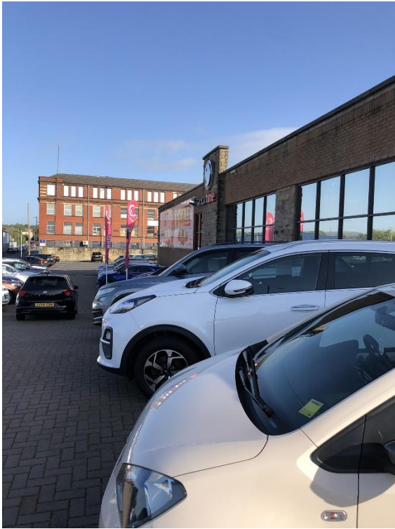
Photograph 1: Overview of the west elevation. Building has brick and stone cladding.
