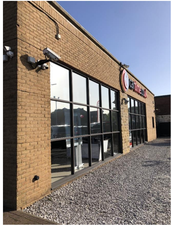
Photograph 3: Overview of the south elevation that fronts Bell Lane.
