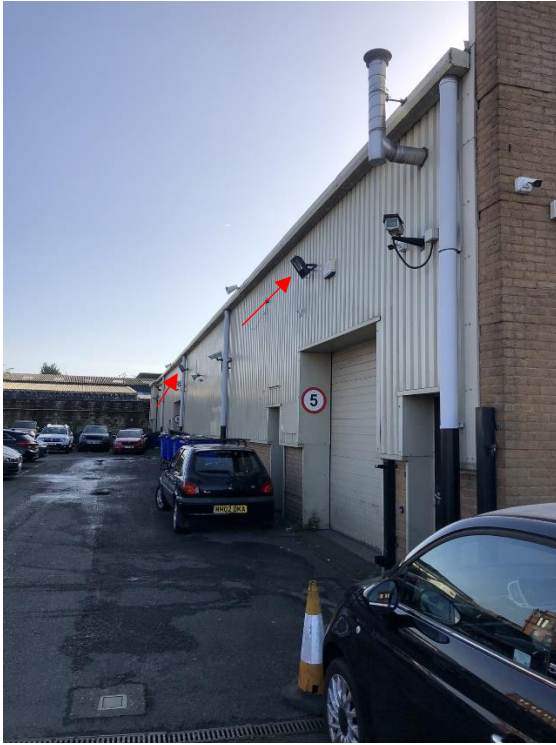
Photograph 5: North elevation (Building 2) which is a service depot. Corrugated metal sheeting and intense security lighting.
