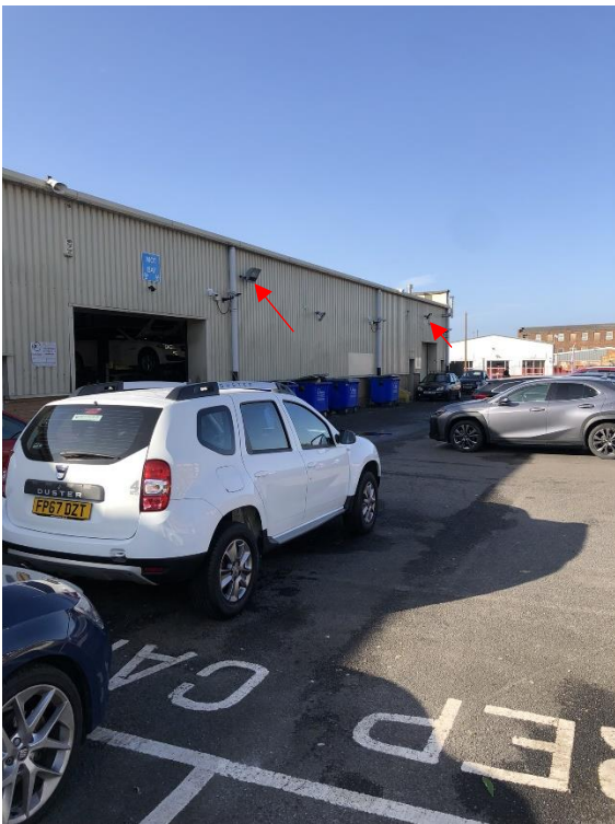
Photograph 6: North elevation of Building 2. High light pollution from security lighting.
