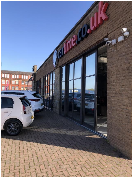
Photograph 2: Overview of the west elevation. Retractable glass doors.
