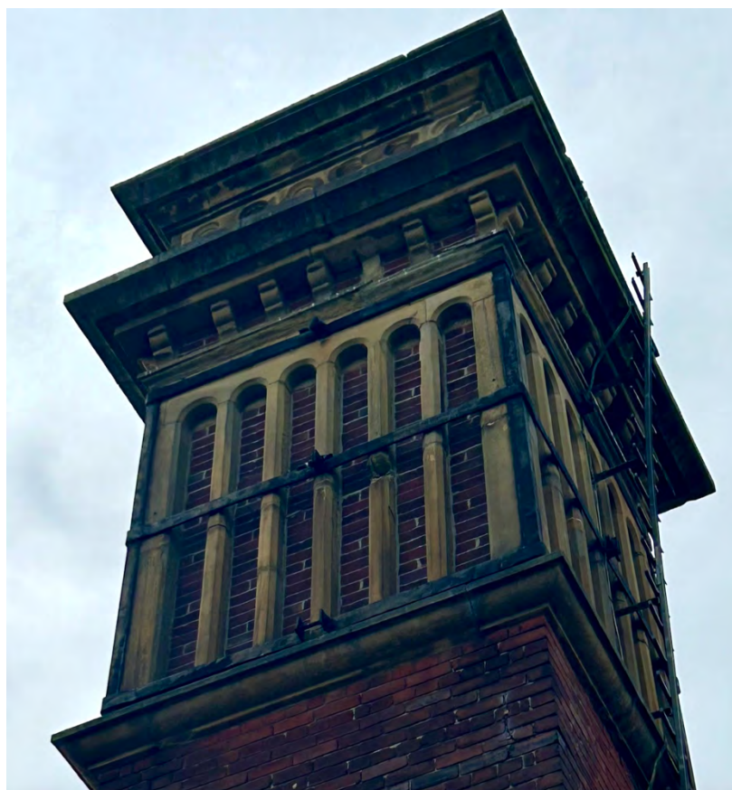
Photo 1 - East elevation of ventilation tower
