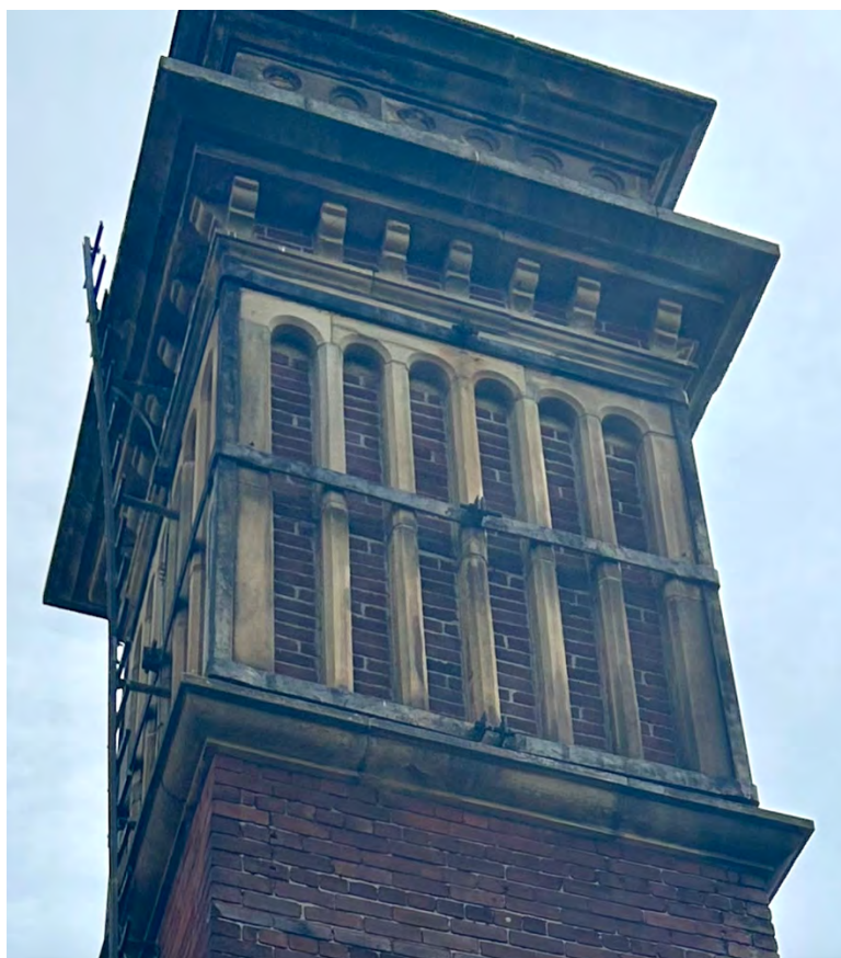
Photo 2 - West elevation of ventilation tower
