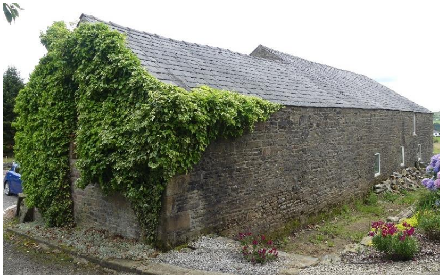
Figure 7: The western elevation of the main western range prior to the change of use works commencing
