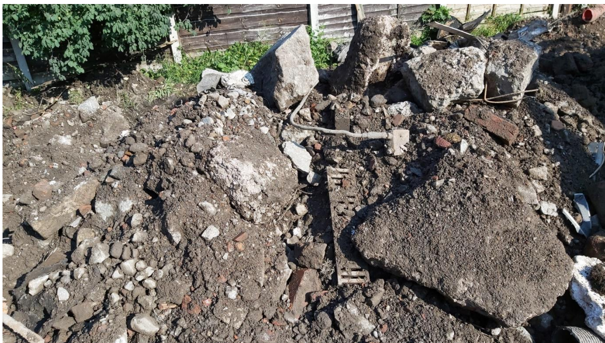
Photograph 11 – Excavated Concrete Hardstanding Stockpiled Prior to be Taken Off Site for Recycling
