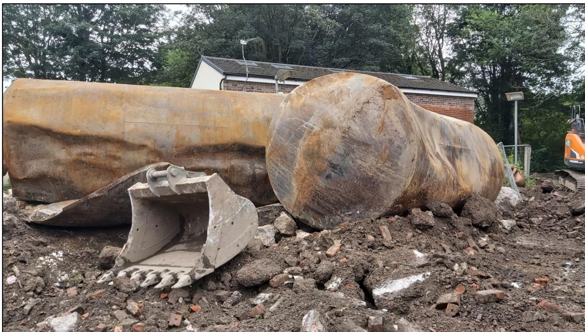
Photograph 8 – Removed Tanks Waiting for Transport off Site
