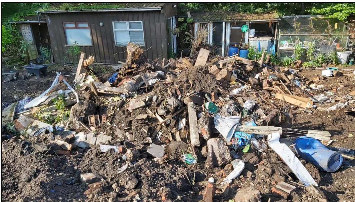
Photograph 10 – Cleared General Waste, Wood, Plastic etc temporarily stored on adjacent site (this site also owned by the developer) prior to disposal off-site
