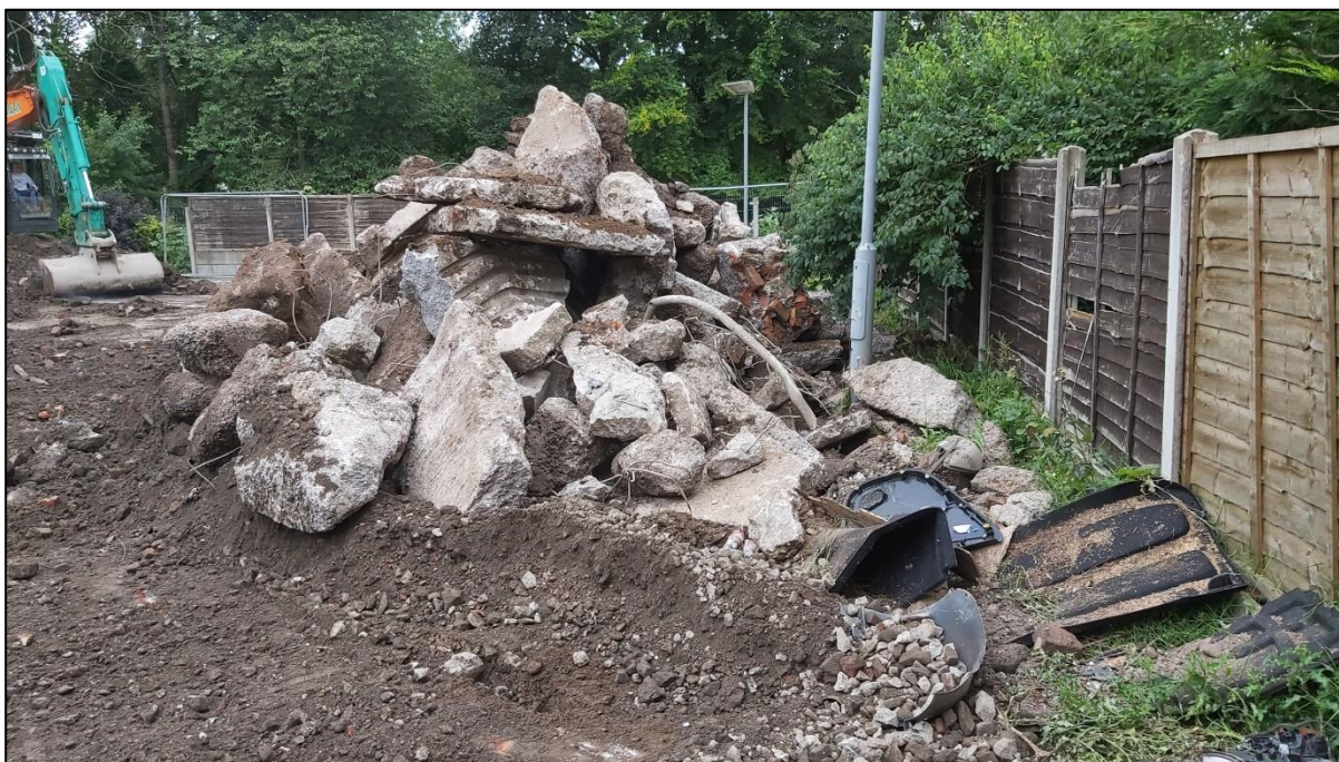
Photograph 7 – Concrete Hardstanding to Be Taken Off Site for Recycling
