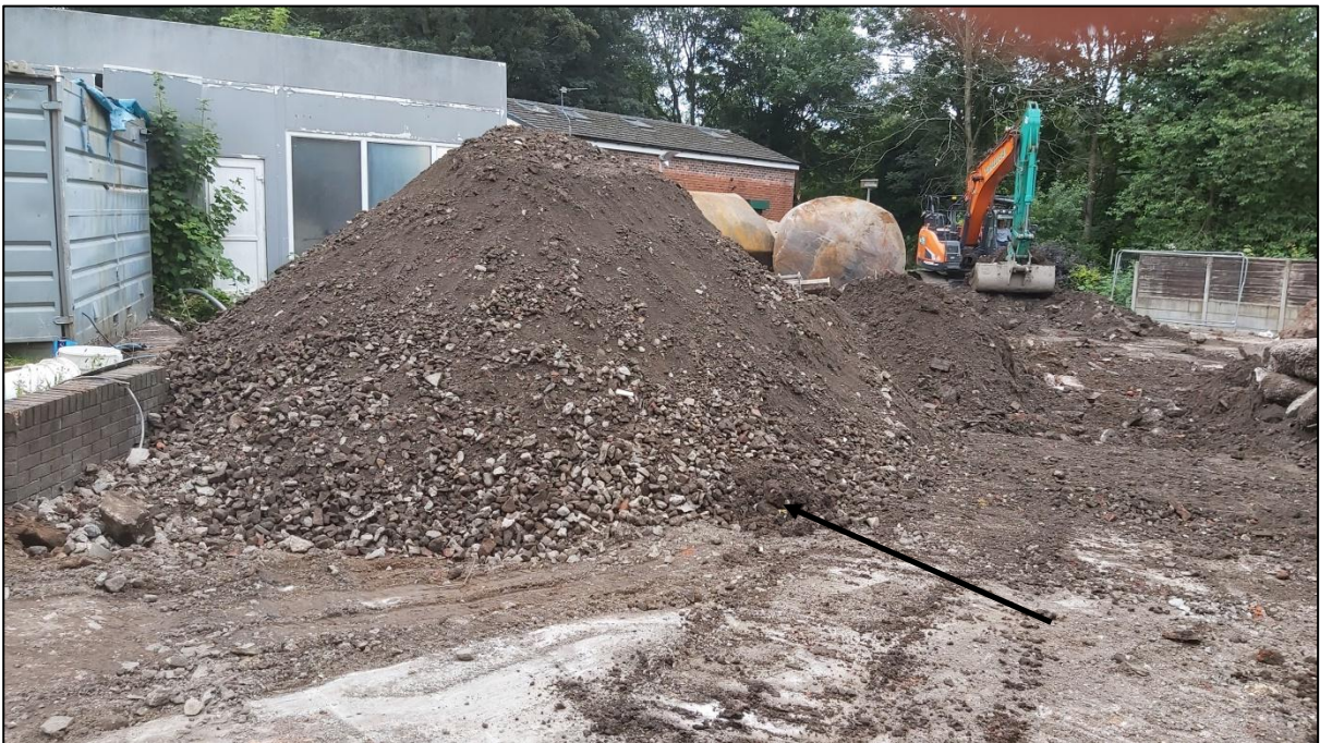
Photograph 6 – Imported 6F2 Used to Backfill Tank Excavations
