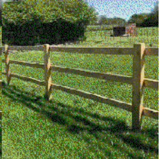
FENCE SURROUNDING SITE
