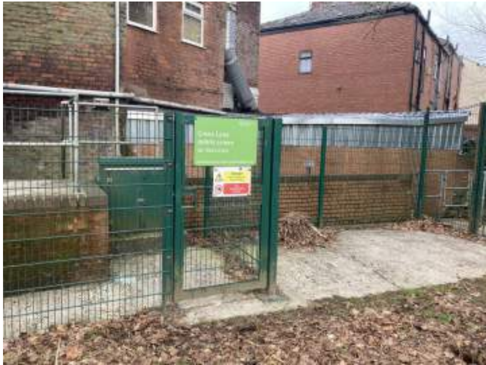
Plate 25 – Cross Lane debris screen, north of site
