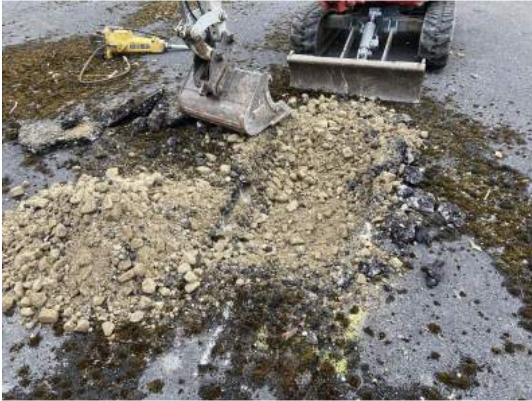
Plate 11 – TP4 gl to approximately 0.2mbgl with arisings
