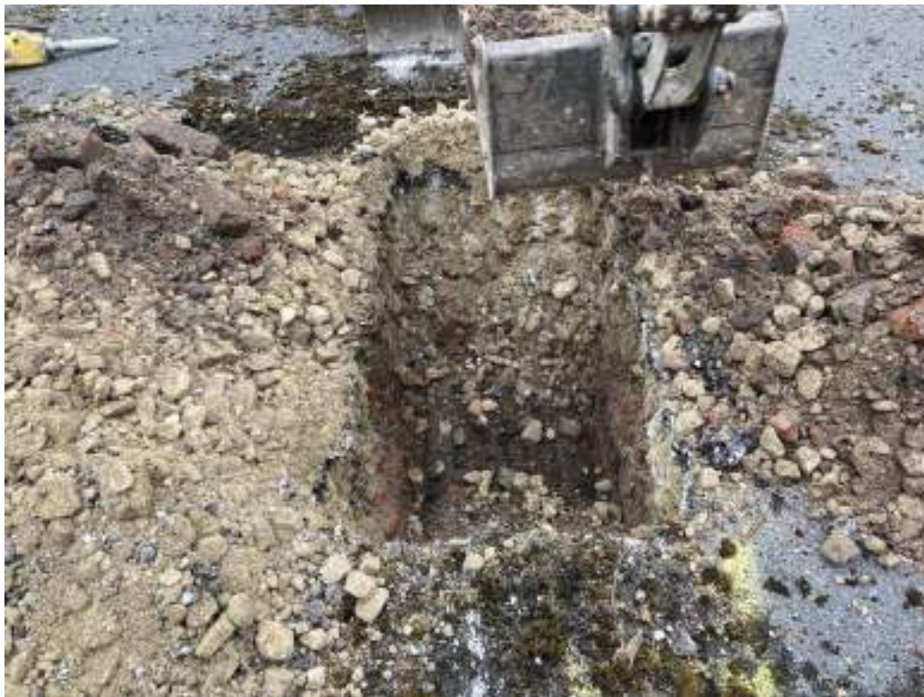
Plate 12 – TP4 gl to approximately 0.4mbgl with arisings
