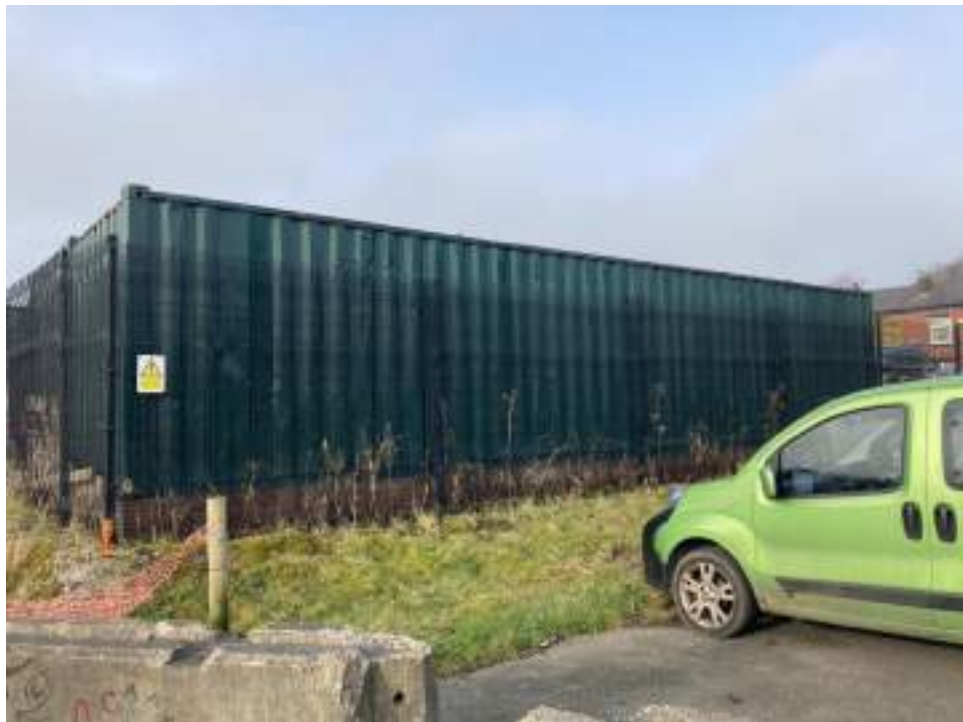
Plate 26 – Japanese Knotweed treatment works south west of site
