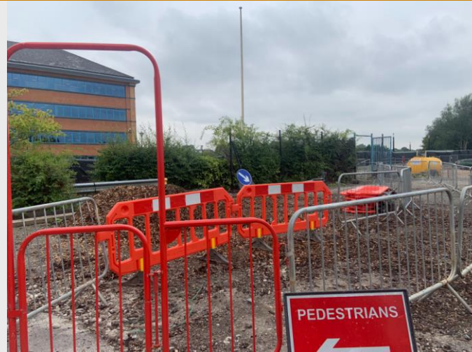
Photograph 2: View of the southeastern hedgerow with construction fencing in front
