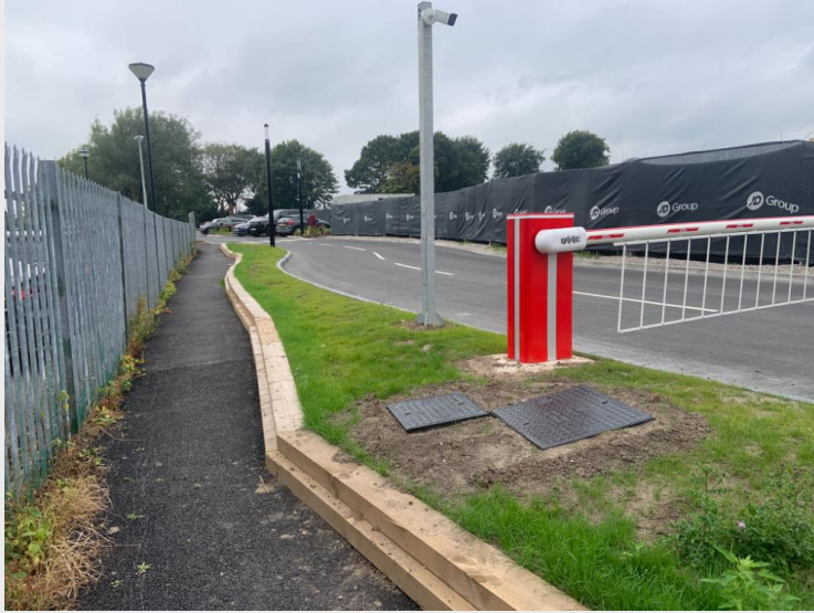
Photograph 9: Southern line of hardstanding pavement with grass
