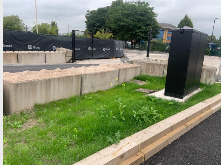
Photograph 10: Southern line of pavement with newly sown grass
