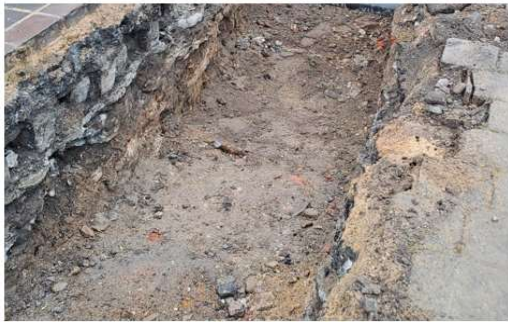
Fig 6 Photos of excavations to demonstrate existing pavement construction
