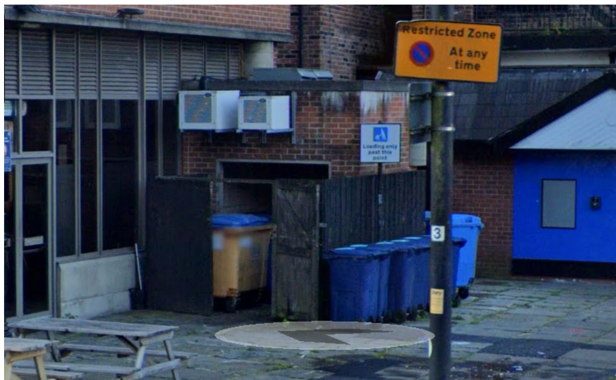
5-10 Market Pl. Outdoor Bin Store (Black coloured timber frame)
