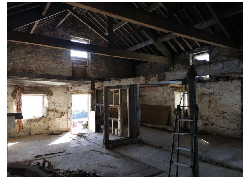
INTERIOR OF BARN
