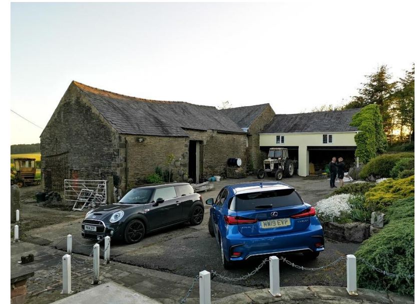
NORTH EAST CORNER OF BARN
