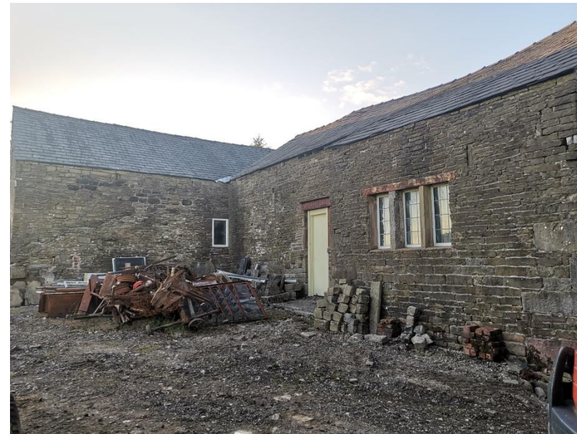
SOUTH WEST CORNER OF BARN
