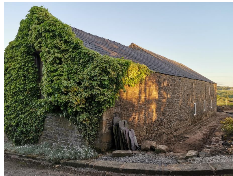
NORTH EAST CORNER OF BARN
