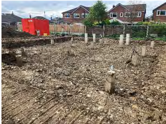
PLATE 7 PILE MAT AND PILE INSTALLATION
