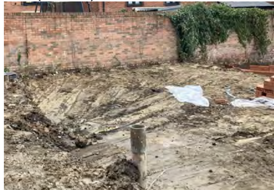
PLATE 11 REDUCED LEVEL DIG TO EXPOSE NATURAL SUBSOIL IN FORMER TENNIS COURT AREA (PLOT 25)
