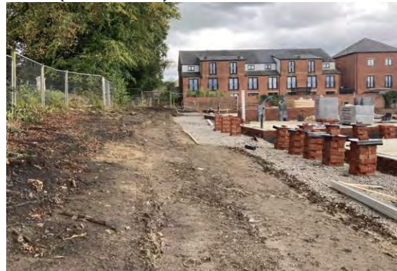
PLATE 12 REDUCED LEVEL DIG TO EXPOSE NATURAL SUBSOIL IN FORMER TENNIS COURT AREA (PLOT 20-24)
