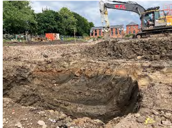
PLATE 8 SOFT CLAY ENCOUNTERED DURING DRAINAGE EXCAVATIONS
