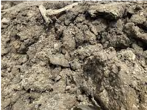
PLATE 9 SOFT/ORGANIC CLAY ENCOUNTERED DURING DRAINAGE EXCAVATIONS
