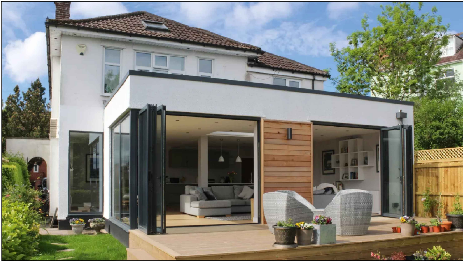
flat roof extension with parapet detailing, patio doors and corner glazing
