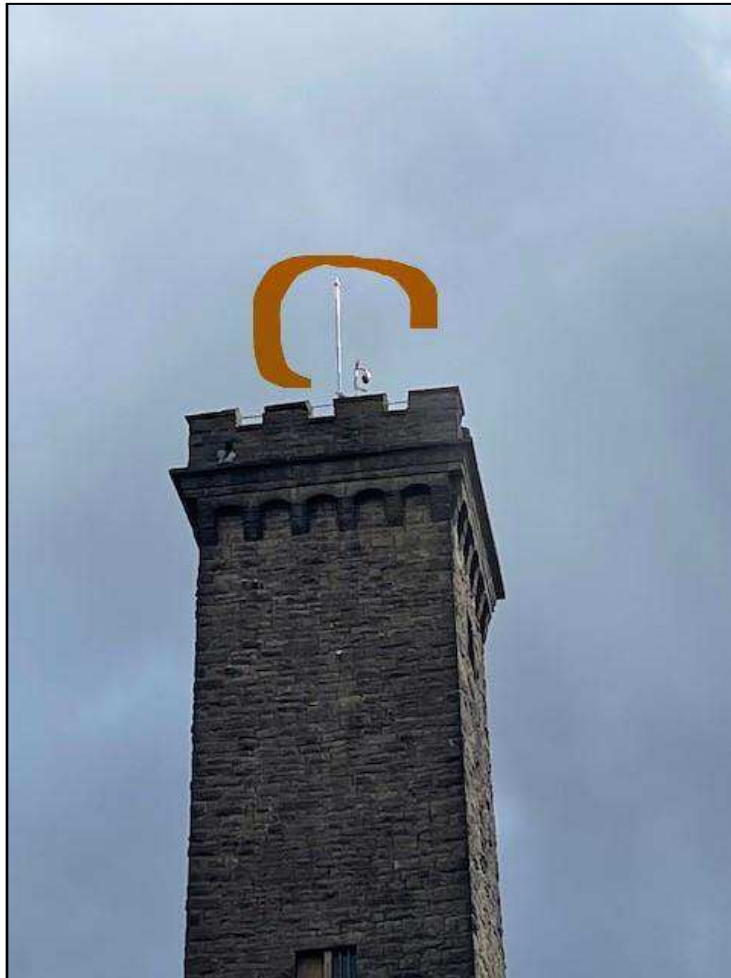
Figure 9: Photo of top of tower with camera equipment visible above battlement parapet
