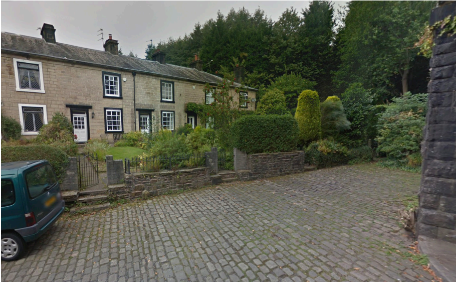
View 1 - Elevation fronting Summerseat Viaduct (in 2015)
