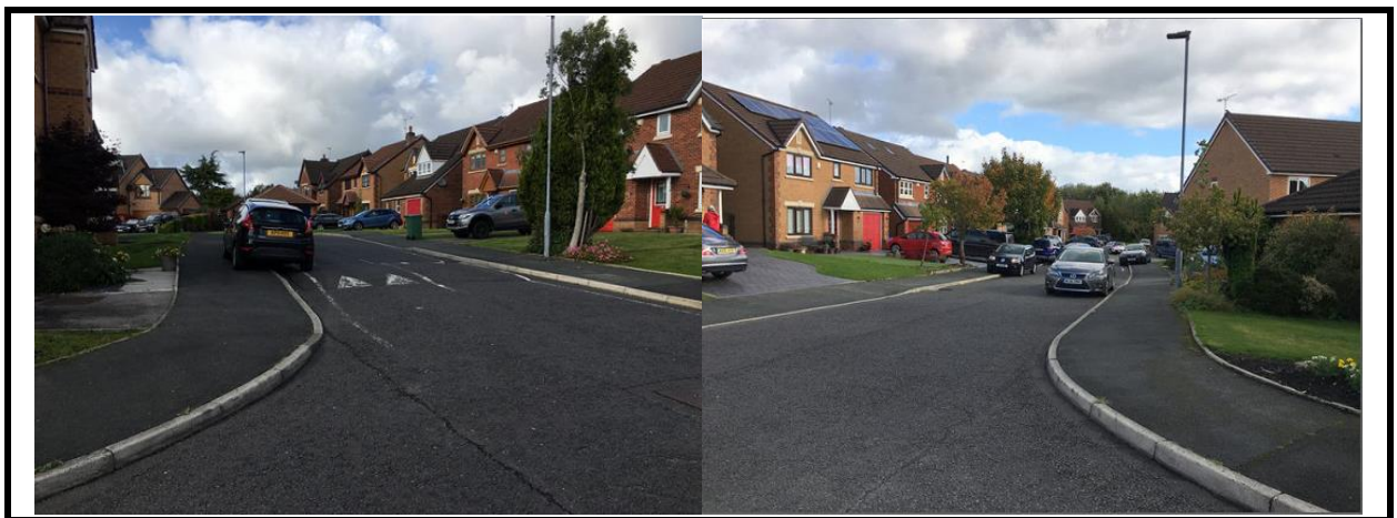
Brownhills Close junction view left and right
