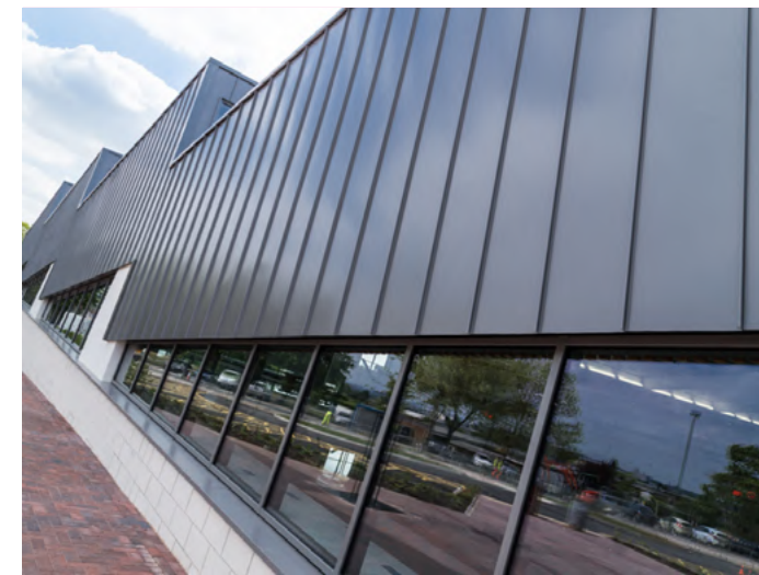
Cladding to the sports hall
