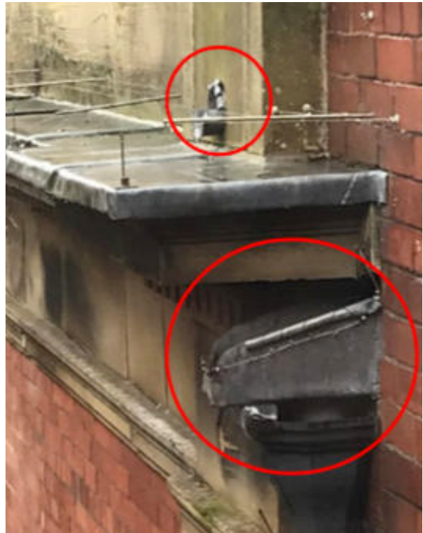
03 (Area C). View from the gutter above. View from the north-west showing the overflow and hopper (circled).
