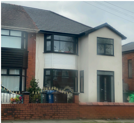
Image 6C - Photo of No. 136 Parkhills Road
