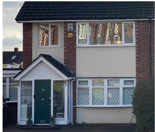
Image 3A - Photo of existing weathered timber porch
