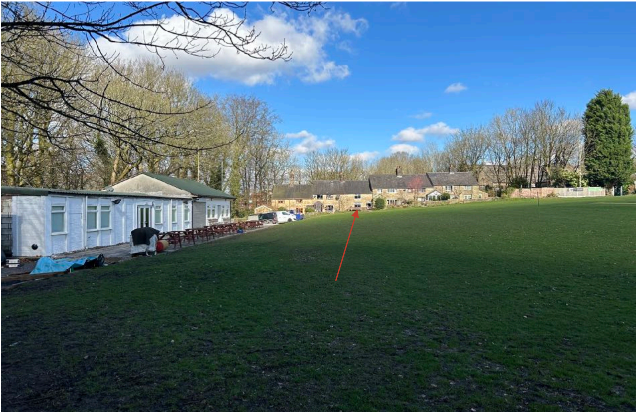
Figure 7: View from far side of cricket pitch. Door/ window indicated. Note that the lower portion of the door is not visible from further afield. Cricket club house pictured left.
