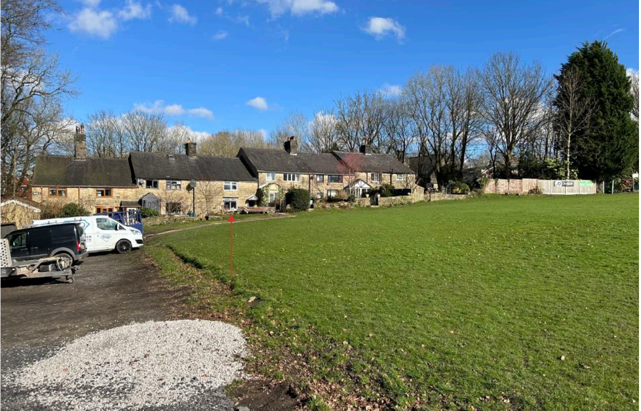
Figure 6: Present day. Proposed door location indicated. Note the extensive modern alteration such as the PVC windows and doors, porches, Velux, concrete and timber panel fencing etc.
