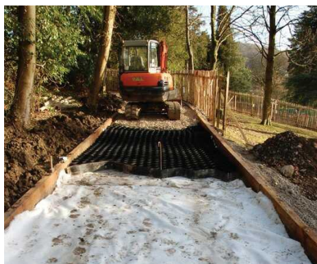
Fallbarrow Park, Windermere: CellWeb TRP® Installation
