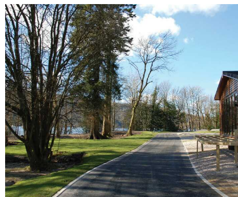
Fallbarrow Park, Windermere: Completed CellWeb TRP® Installation
