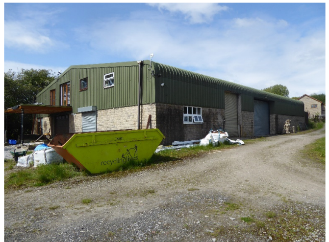
General view of SE/NE elevation.
