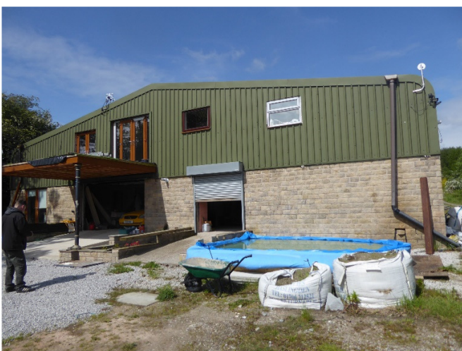
General view of SE elevation.
