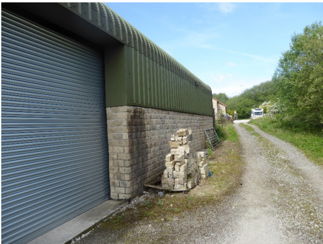
General view of NE elevation.
