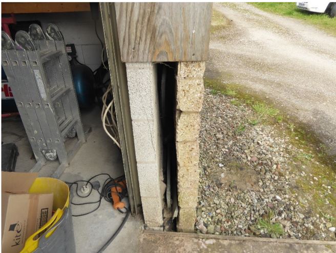
Detail showing building wall cavity.
