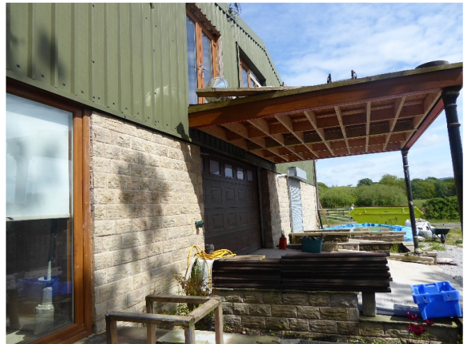
General view of SE elevation.
