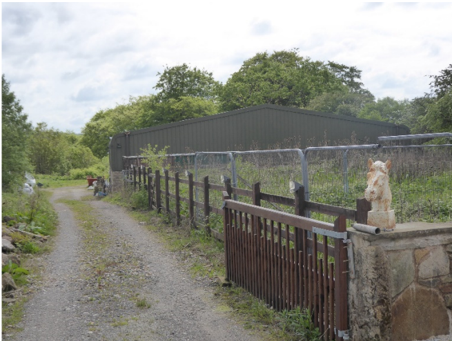
General view of NW elevation.
