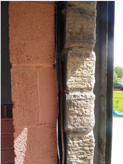
Detail showing building wall cavity.
