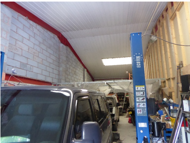
Typical internal area, roof is steel sheeting with no loft space /cavity.
