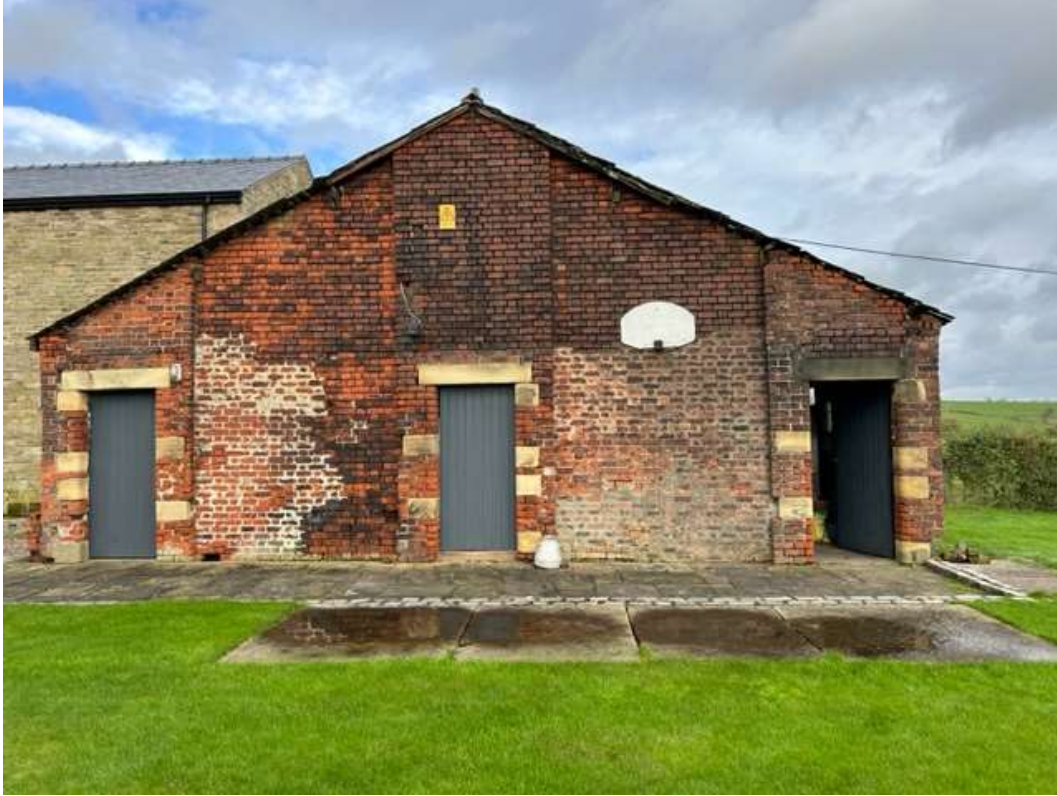
Image 7 – Front elevation of brick shippon
