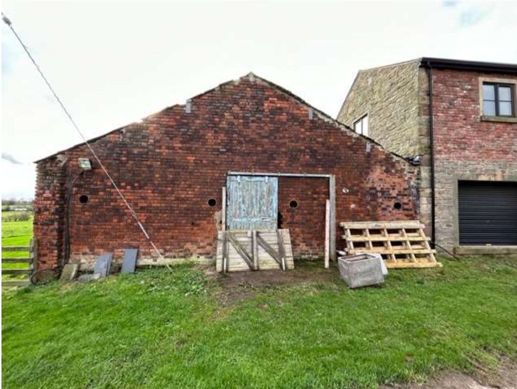
Image 9 – Rear (north) elevation of brick shippon
