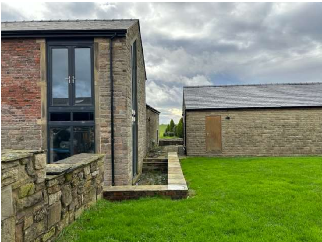
Image 12 – View to rear corner of long barn and detached garage
