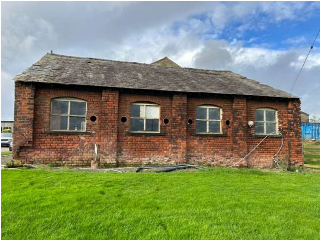
Image 8 – Side (east) elevation of brick shippon
