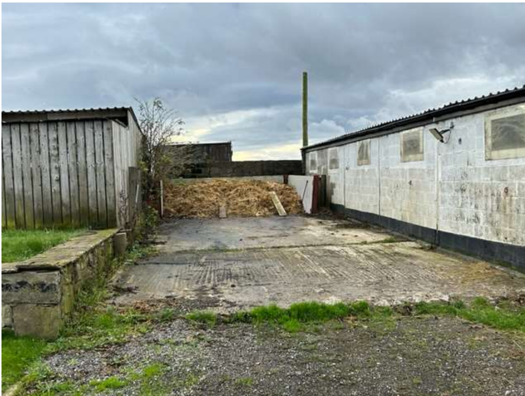
Image 14 – Concrete midden between block stables and agricultural building
