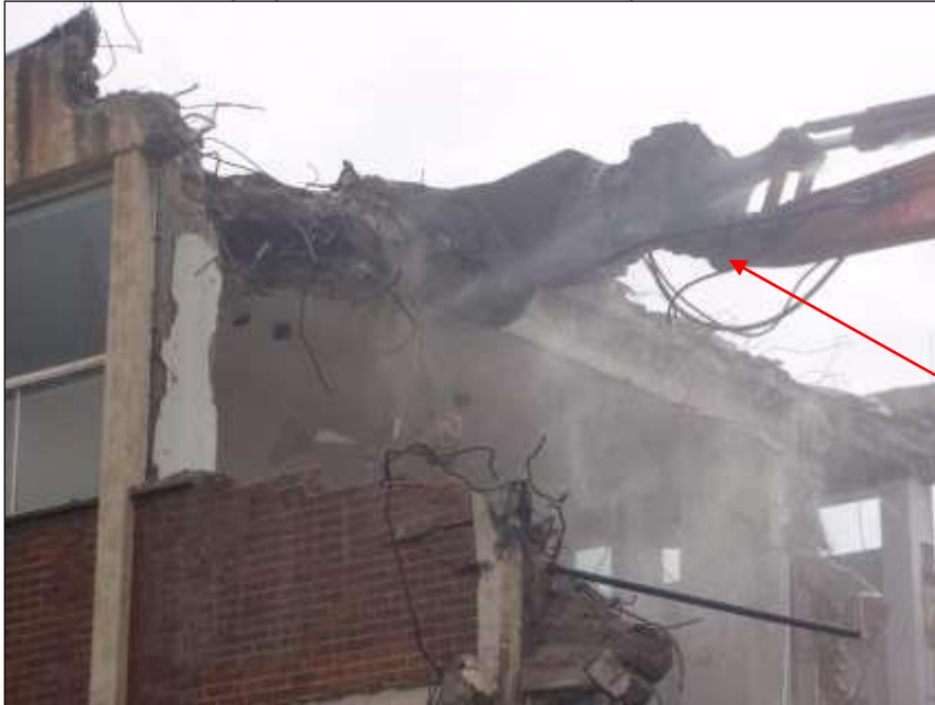
Dust suppression at source
