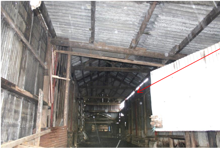
Building 4a - Internal
