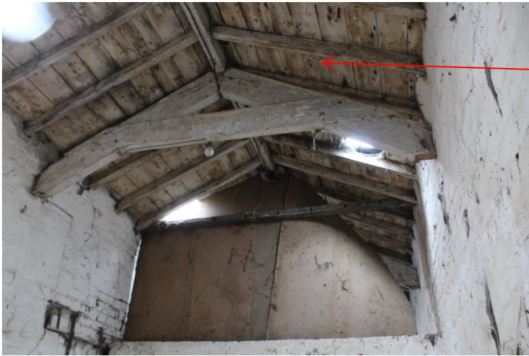
Building 3a - Internal
