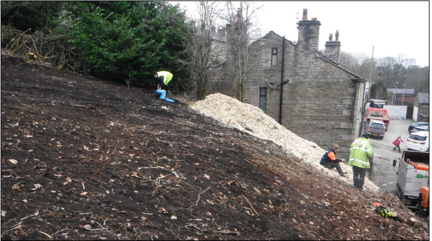
General Site photo viewed north along Tanners St.
