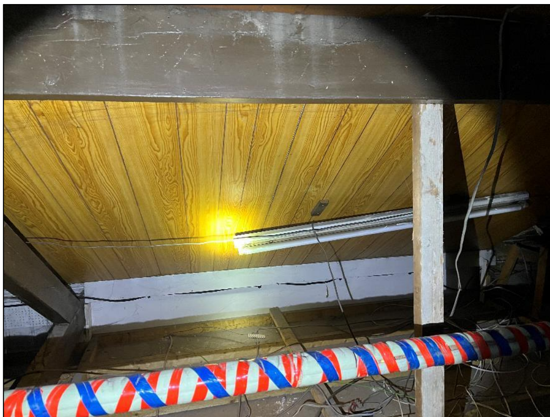
Plate 4 – Timber boarding beneath roof tiles within loft space
