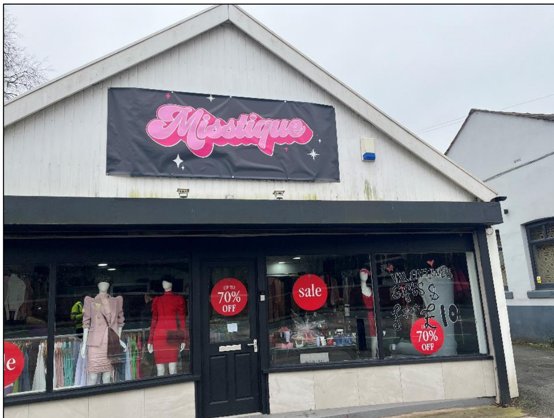
Plate 3 – Shop front at 211 Bury Old Road (eastern aspect)
