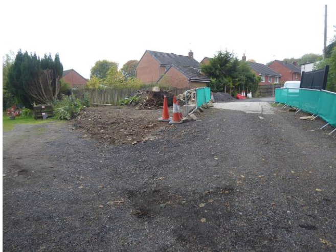
Looking west into the site from the eastern boundary.
