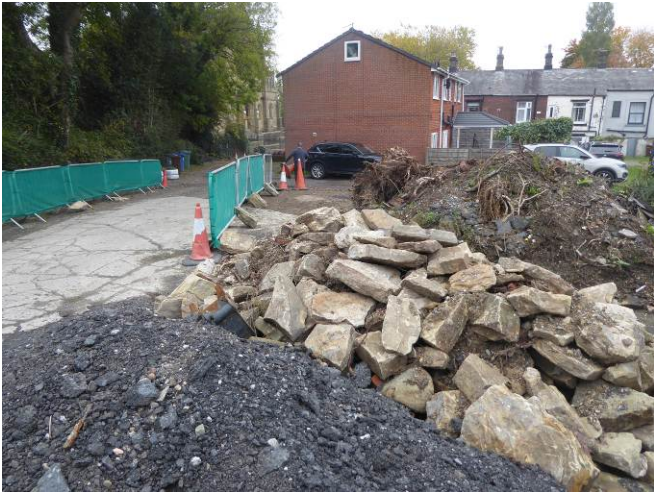
Rubble and spoil mound in the centre of the site.
