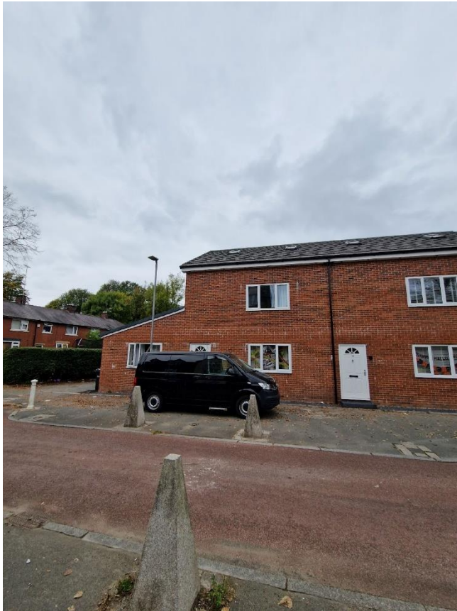
Fig.1: Front of the house
