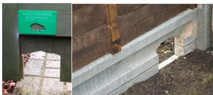
Insert 3: Showing wildlife access gap within fencing
