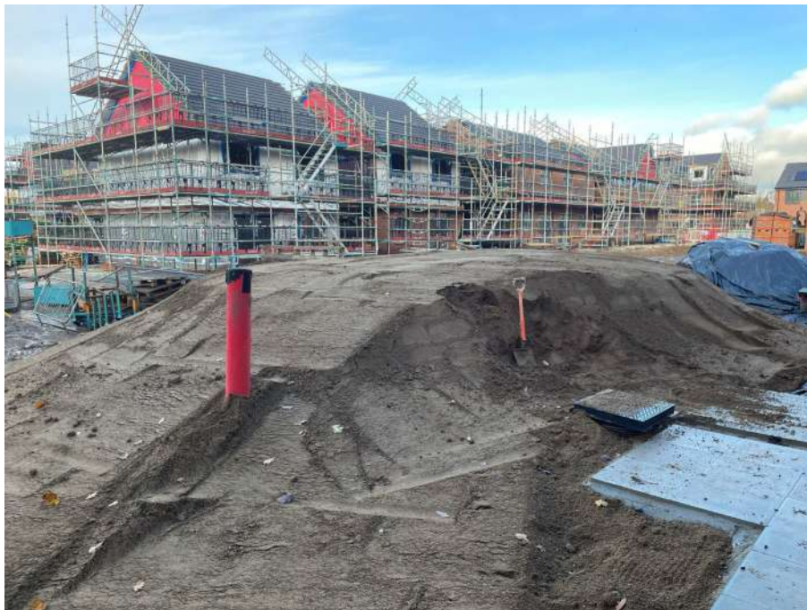
Photographs of SP05 Subsoil Stockpile
