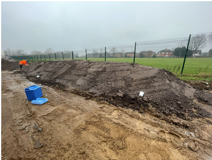
Photographs of SP08 Topsoil Stockpile
