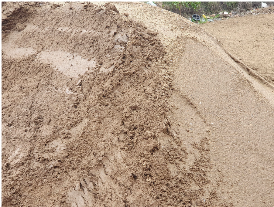
Photographs of SP07 Subsoil Stockpile
