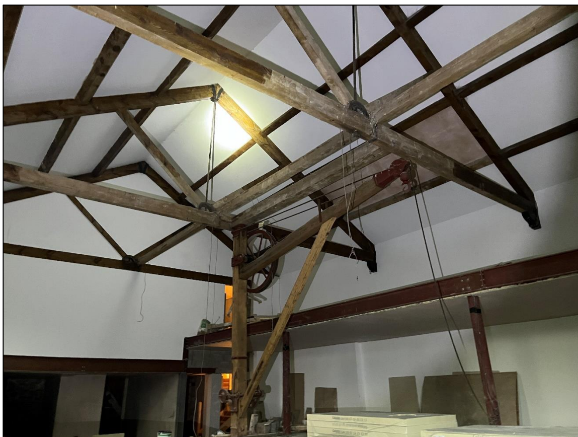
Plate 10 – Internal character of the structure, with obvious signs of renovation
