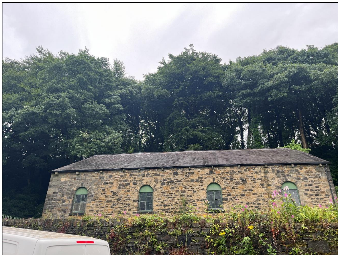
Plate 3 – Western elevation of the Engine Room
