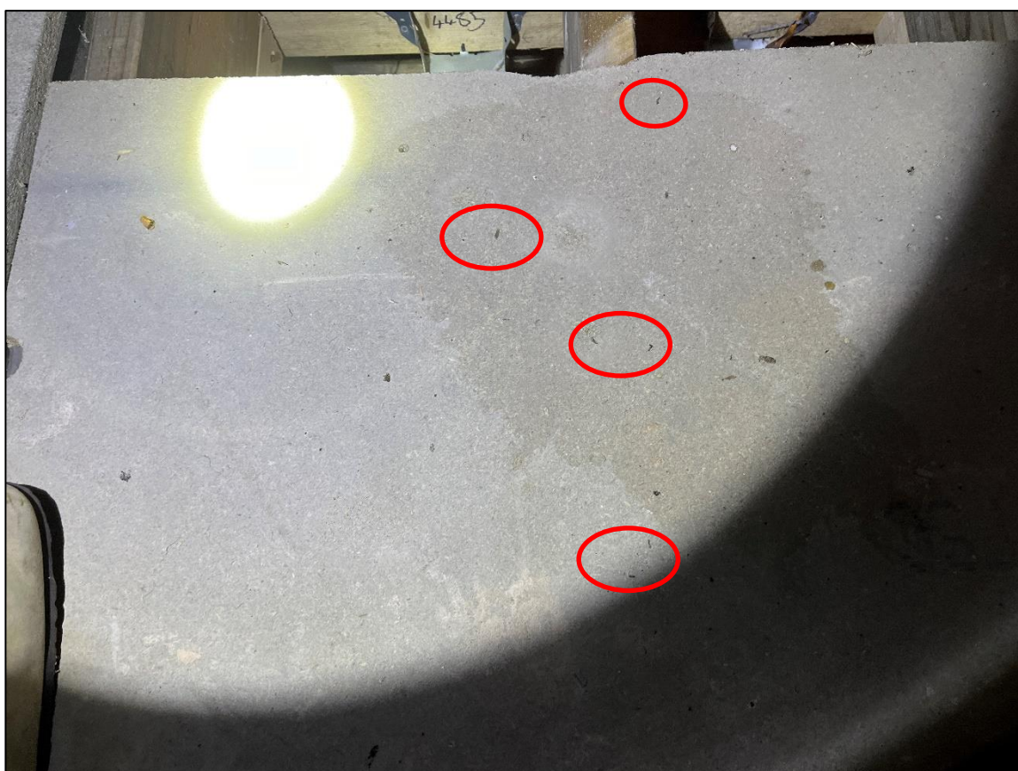
Plate 12 – Example of scattered Pipistrellus droppings within building
