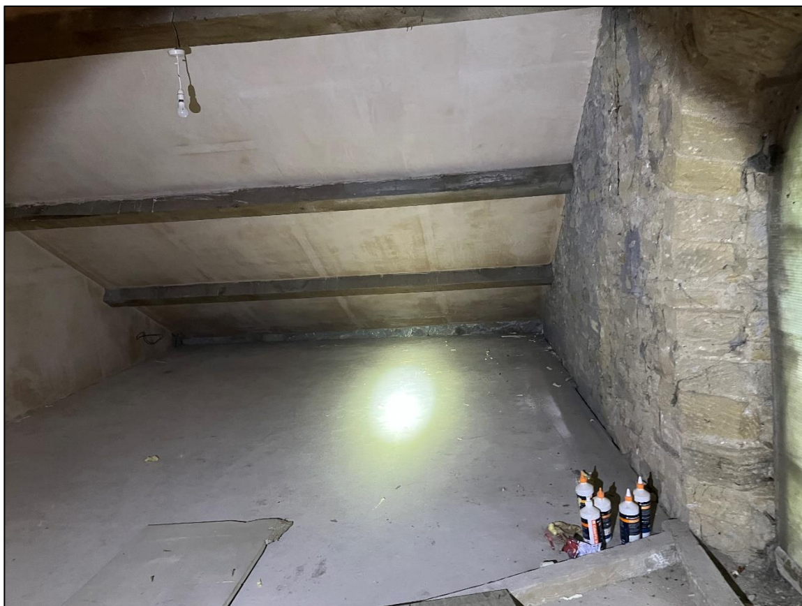
Plate 11 – Nature of mezzanine floor, with plastered roof lining
