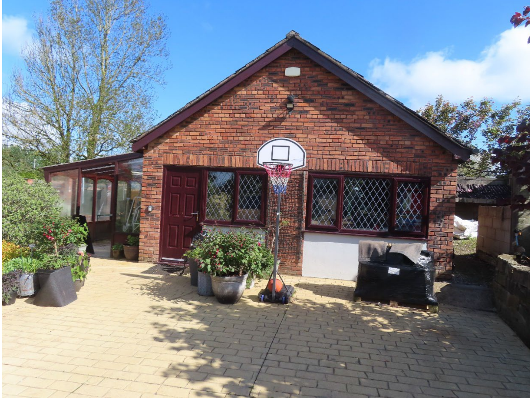
Front elevation of garage converted to annex with lean to summer house.
