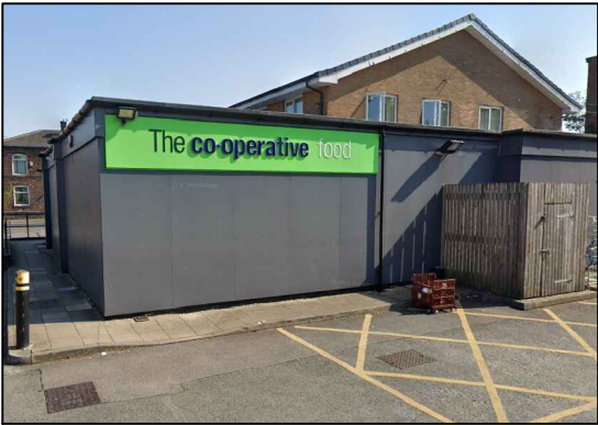
PHOTOGRAPH OF EXISTING ELEVATION A
