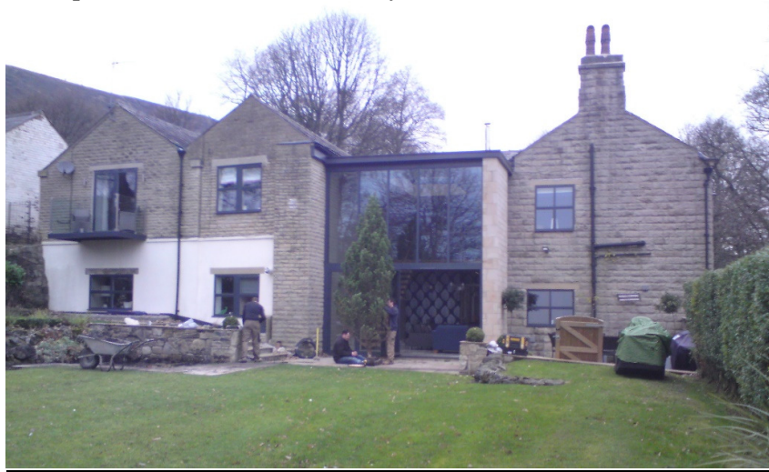
2013 photograph following major renovations
