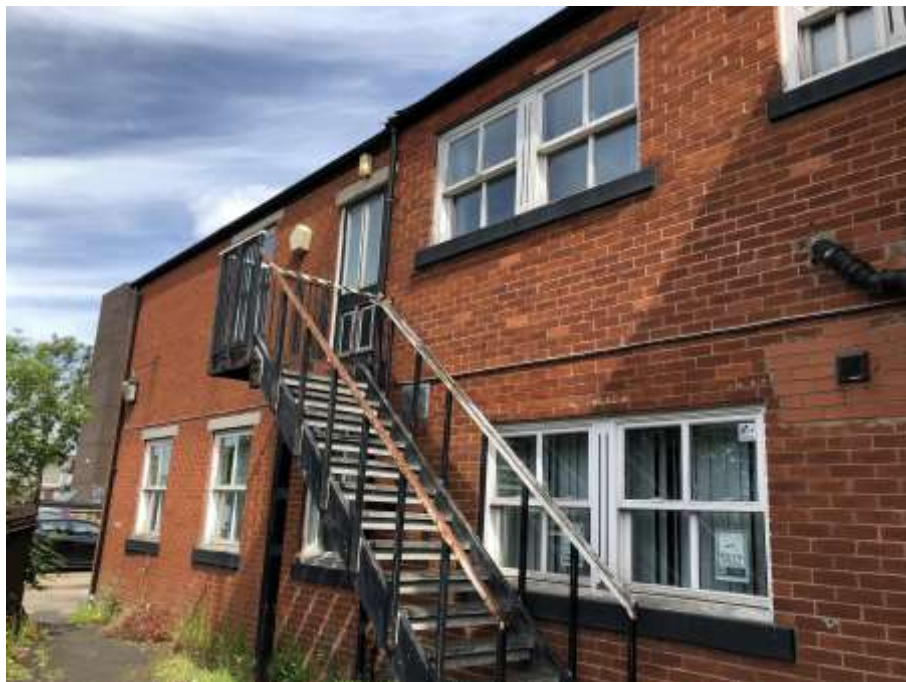
Image 2 – Side elevation (west) and external fire escape/stairs
