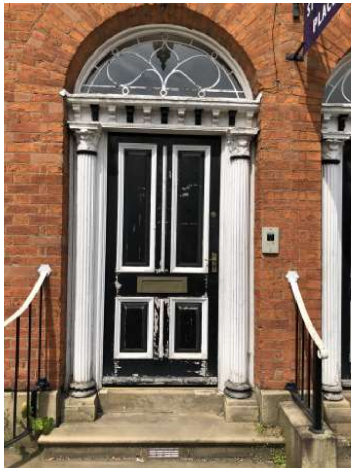
Image 4 – View of existing front entrance door (No 20)
