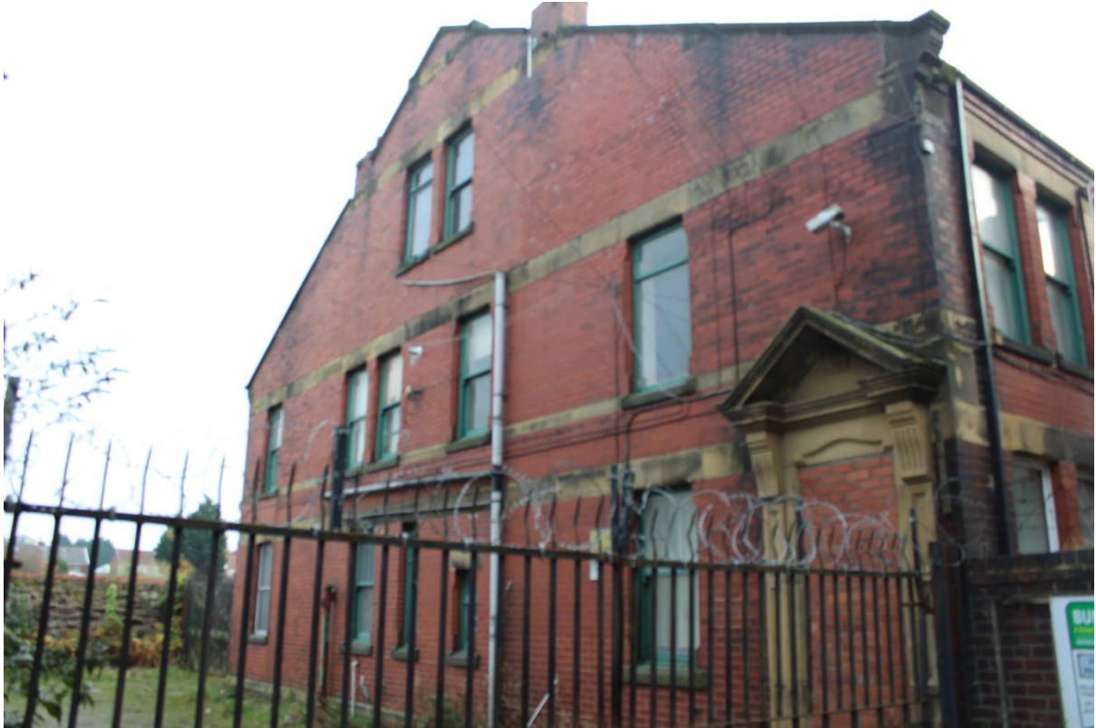
Plate 33 – Albion House North Elevation
