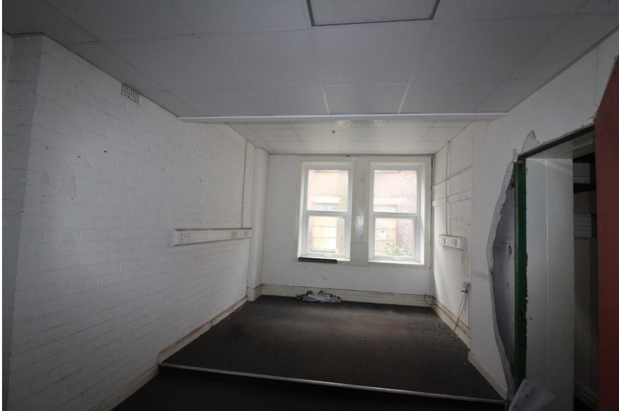
Plate 45 – Ground Floor Offices
