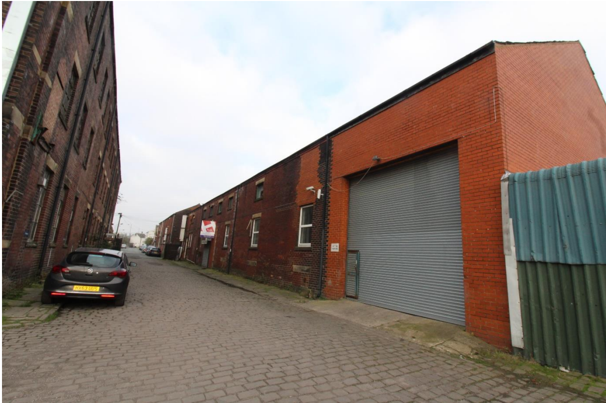
Plate 36 – Albion House West & South Elevation
