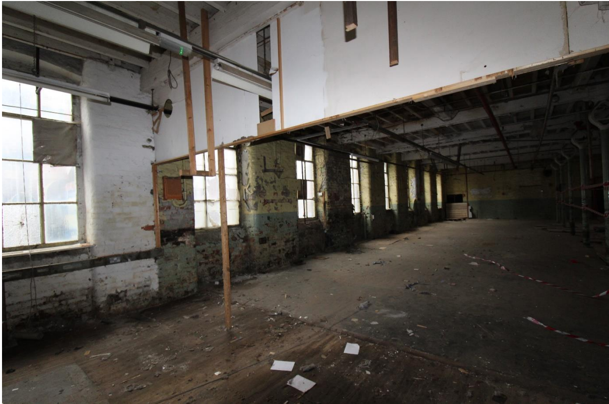
Plate 12 – Ground Floor Original Range
