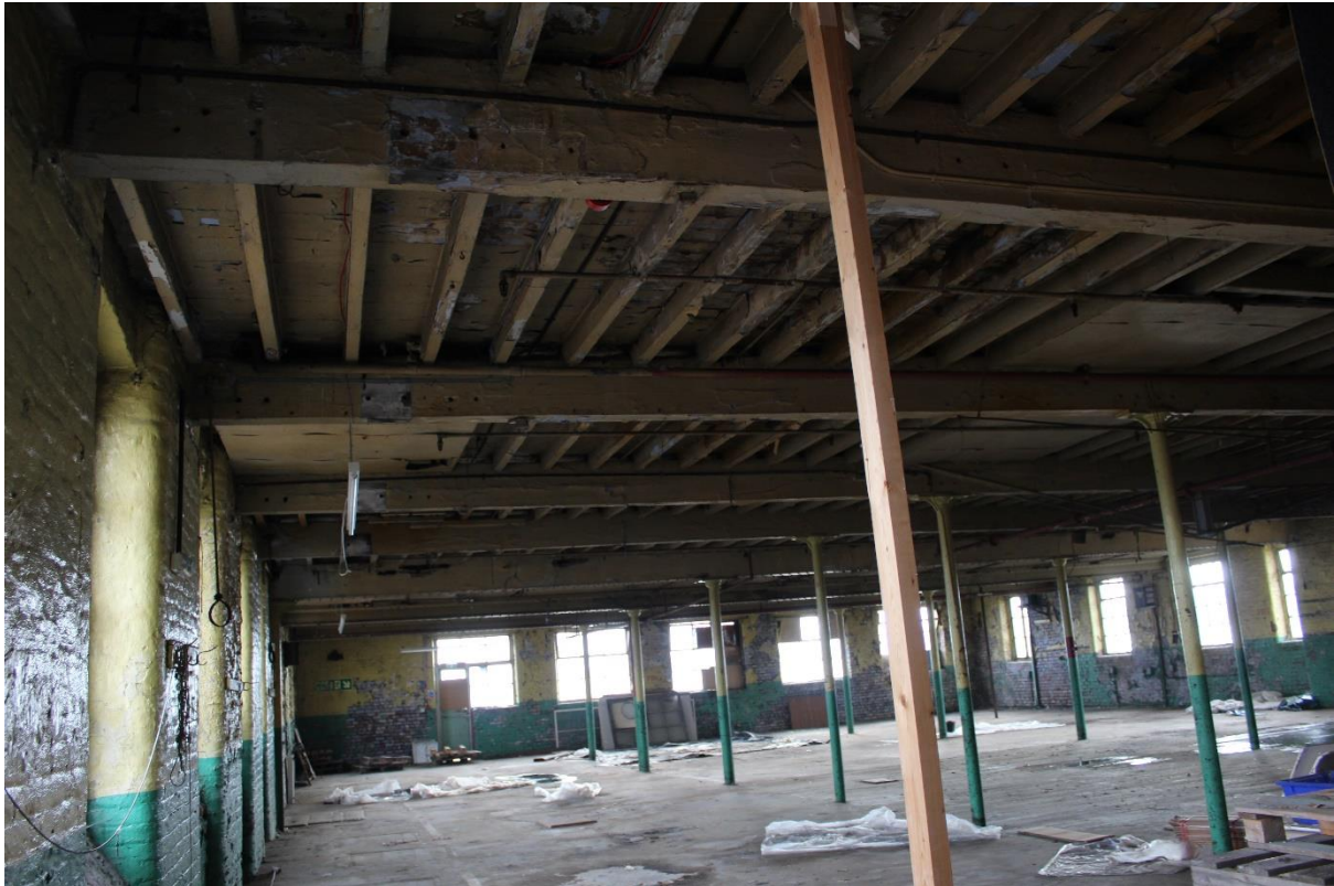
Plate 21 – 2 nd Floor Original Range
