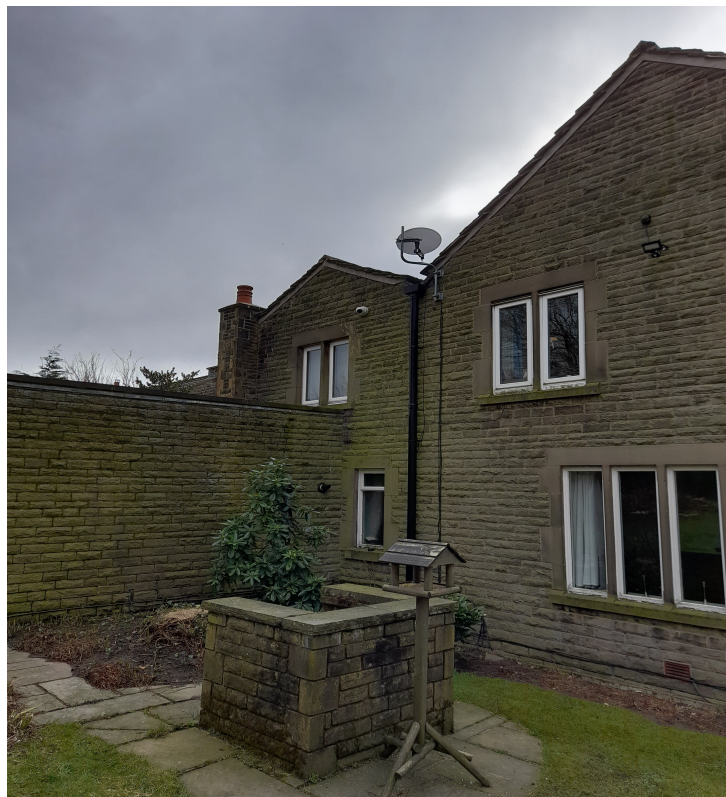
View of part northern elevation.
