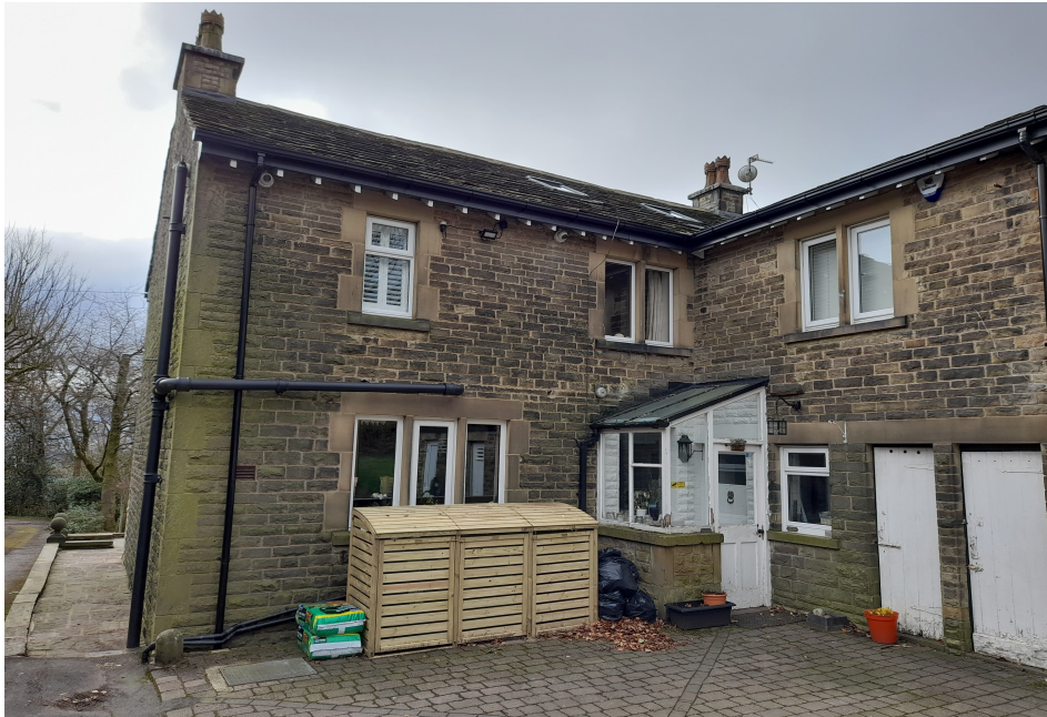
view of existing part northern elevation .
