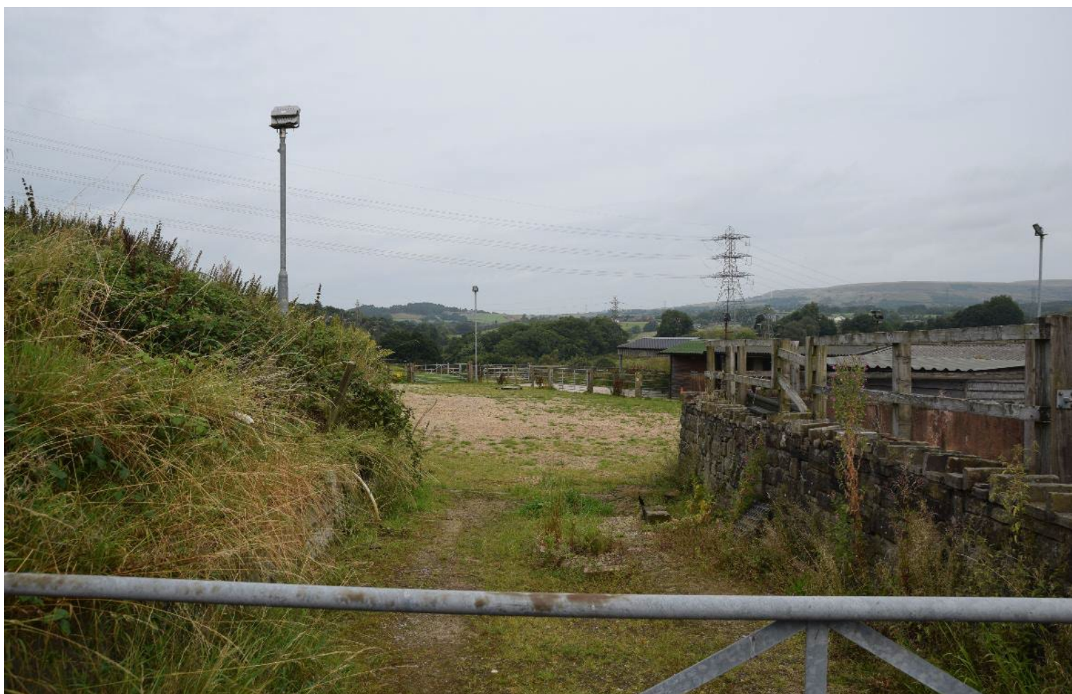
Photograph 6: paddock to the west of the outbuildings, with the stables visible to the north (facing north-)
