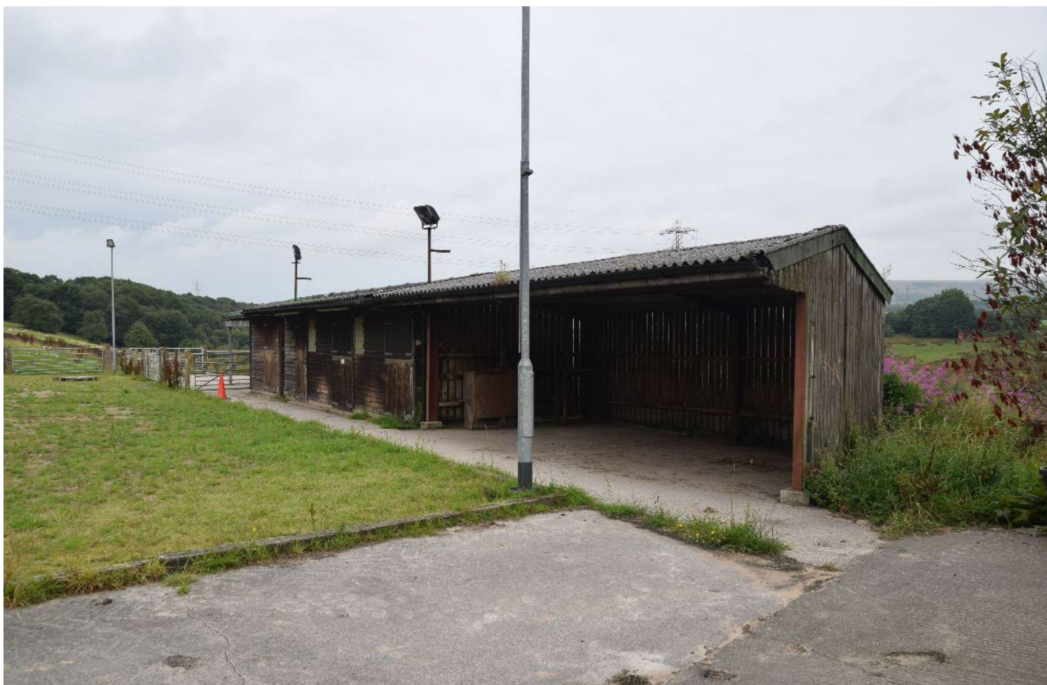
Photograph 10: stables in the west of the Site (facing north-west)
