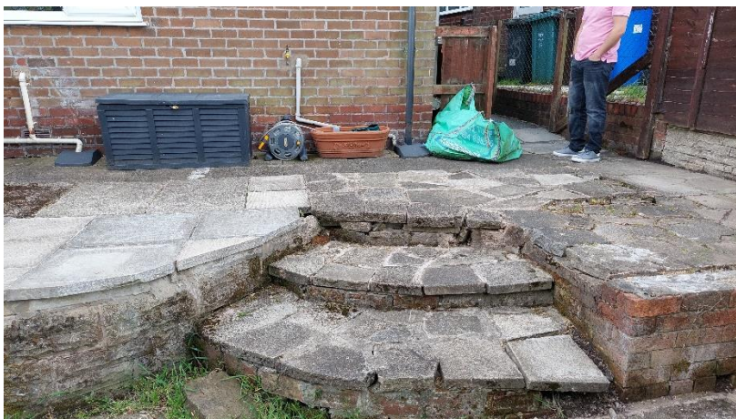
Photograph 3: Stone steps/patio to be dismantled under the close supervision of licensed great crested newt ecologist.
