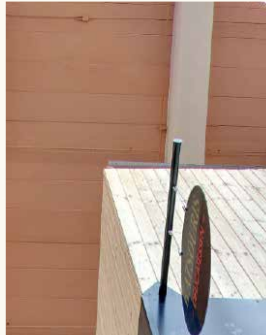
TIMBER FEATURES Meat and Fish Market Interior Ceiling
