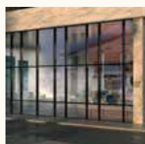
PPC aluminium double glazed curtain wall finished in black RAL9005
