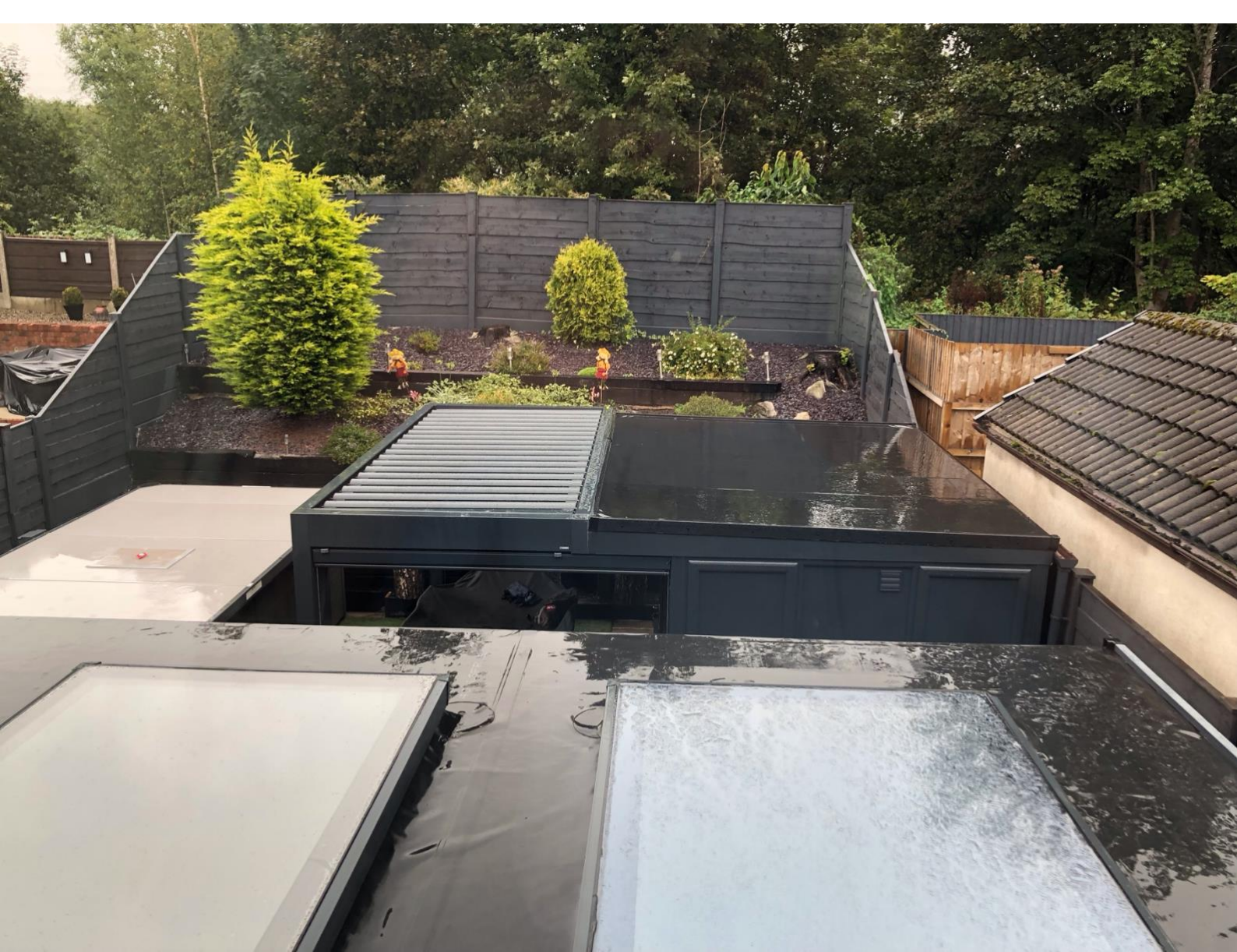
TERRACE PRE DECK SHOWING BOUNDARY AT N033 & 37
