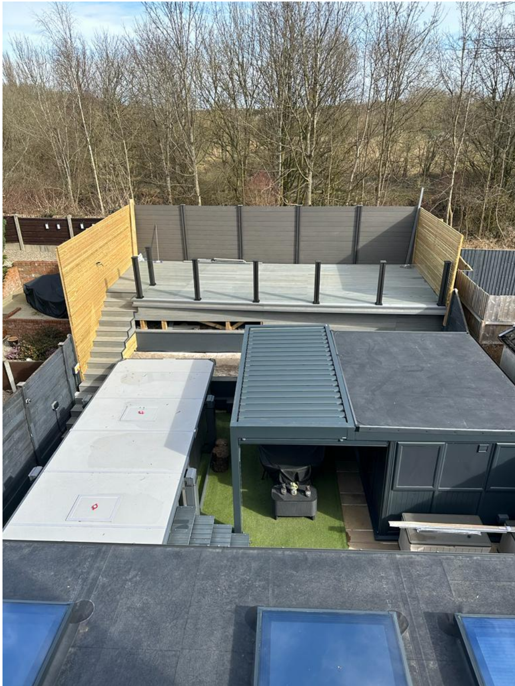
DECK DURING CONSTRUCTION
