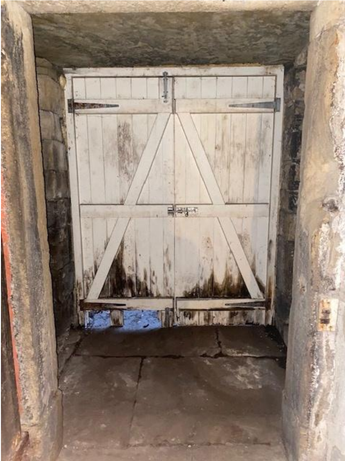
Rear cellar door. Existing-condition photograph for cross-reference with the submitted window and door schedule.
