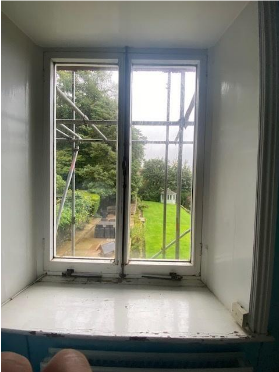
Internal view. Existing-condition photograph for cross-reference with the submitted window and door schedule.
