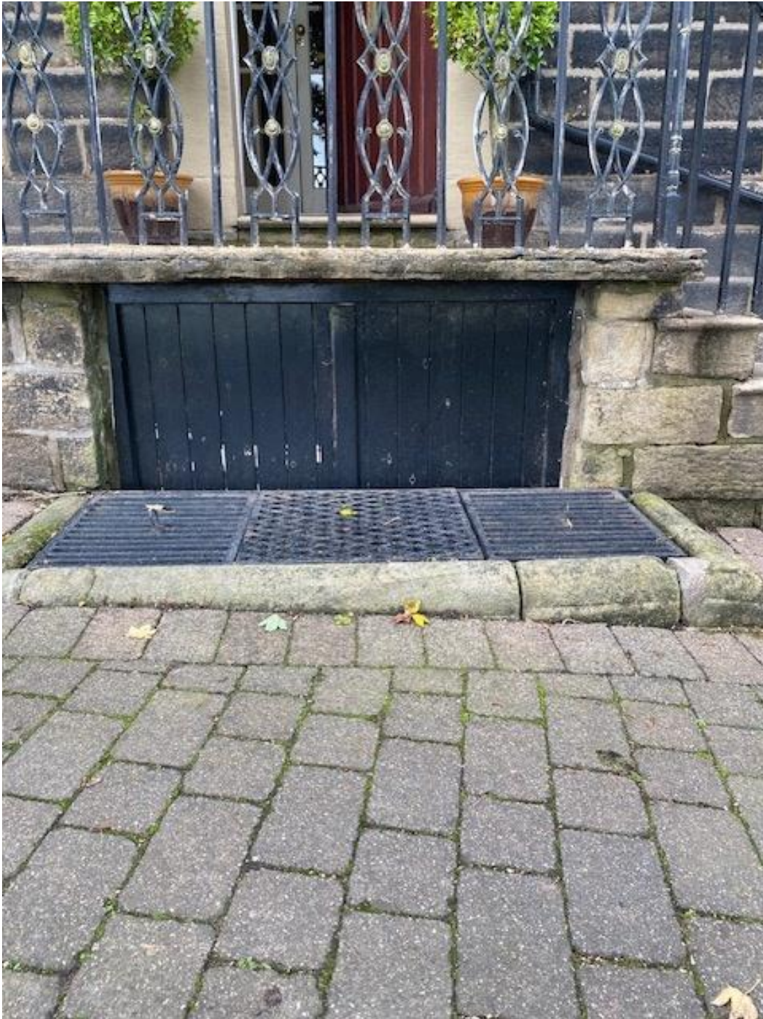
Front cellar door. Existing-condition photograph for cross-reference with the submitted window and door schedule.
