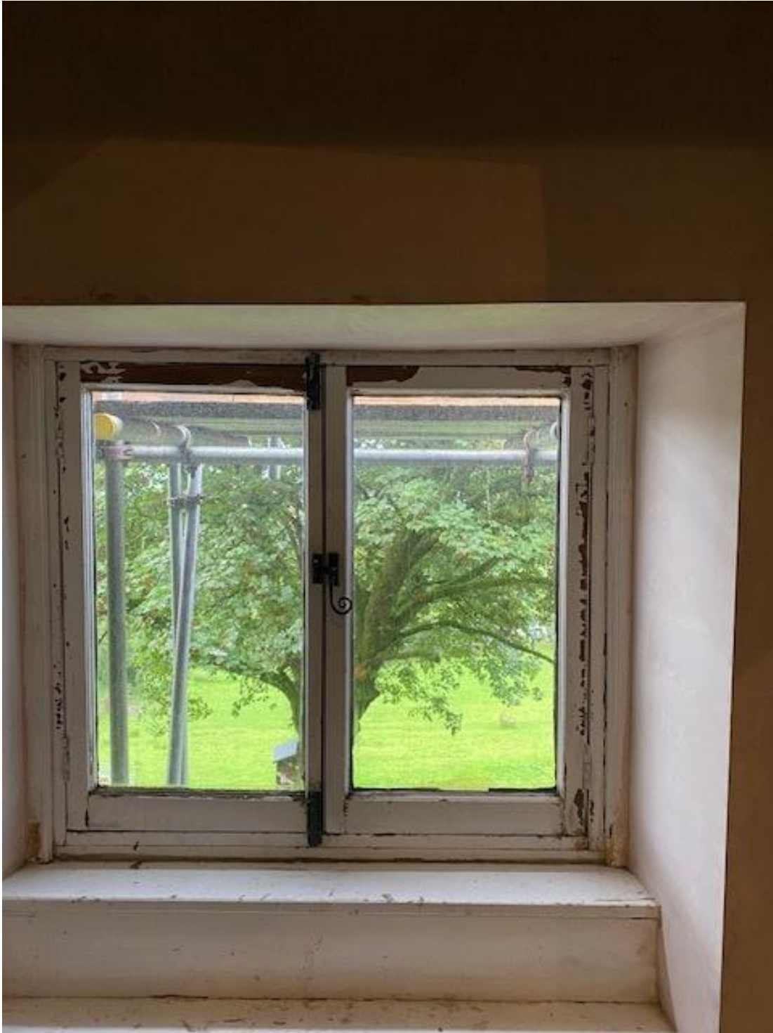
External view. Existing-condition photograph for cross-reference with the submitted window and door schedule.
