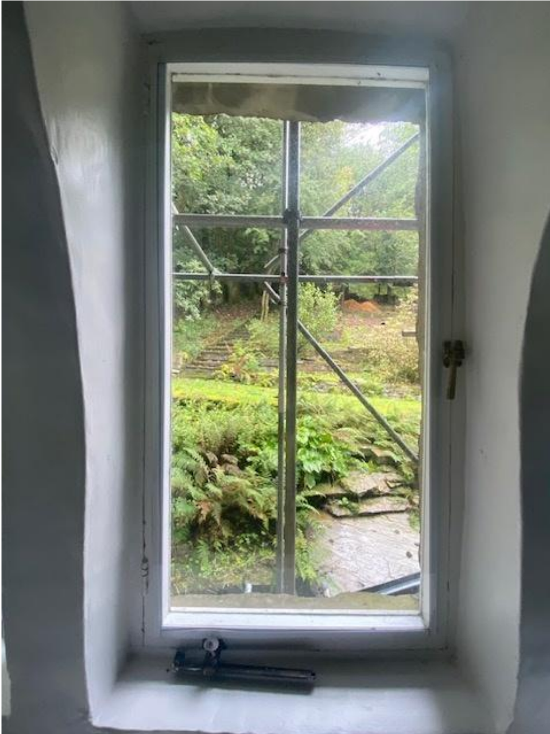
Existing window view. Existing-condition photograph for cross-reference with the submitted window and door schedule.
