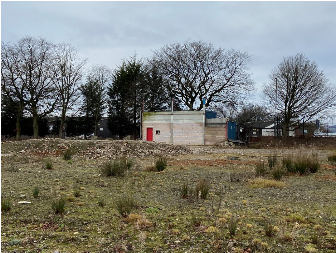
Photograph 5 – Existing building on site.
