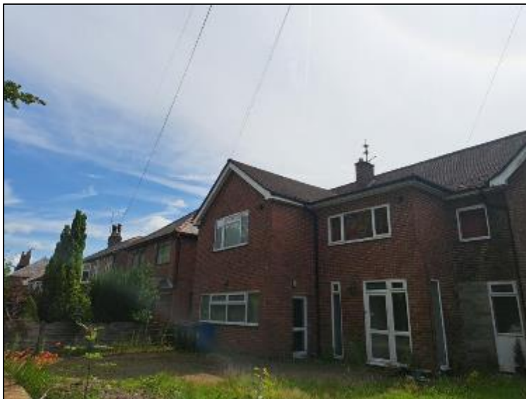
Photograph 1. Showing the front elevation of the building.
