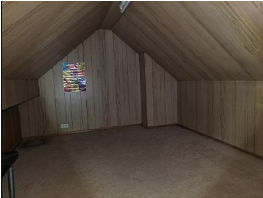
Photograph 9. Showing a different section of roof void in the building.
