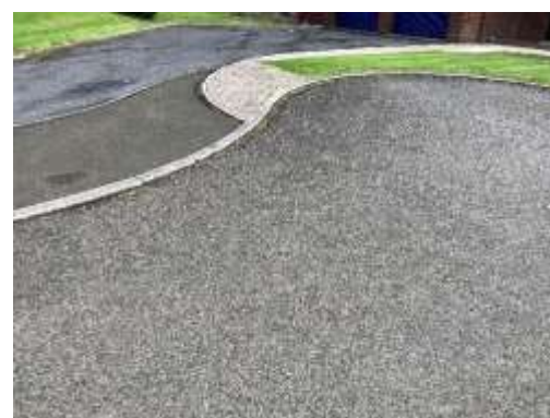
Eastbound (Looking NE) – chainage 40
