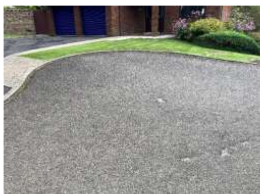
Eastbound (Looking NE) – chainage 40
