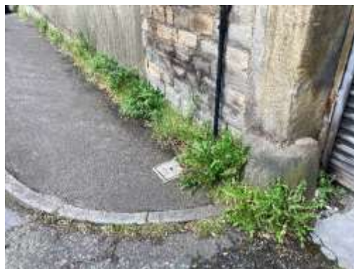
Southbound (Looking Down) – chainage 95
