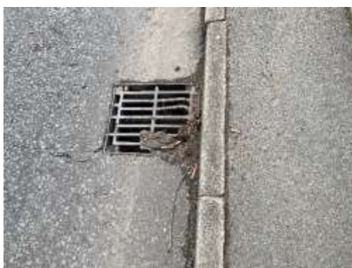
Southbound (Looking Down)– chainage 23
