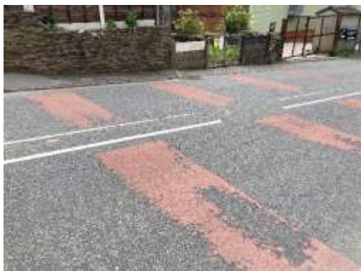
Southbound (Looking SE) – chainage 75
