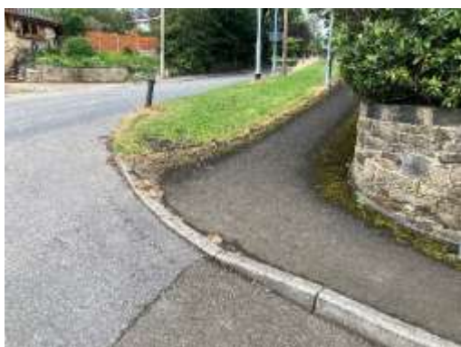
Eastbound (Looking NW) – chainage 8
