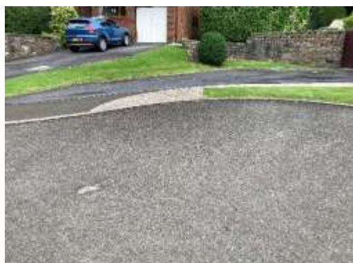
Eastbound (Looking North) – chainage 40
