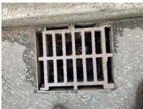
Southbound (Looking Down) – chainage 52
