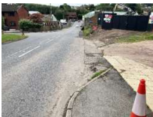
Southbound (Looking South)– chainage 25
