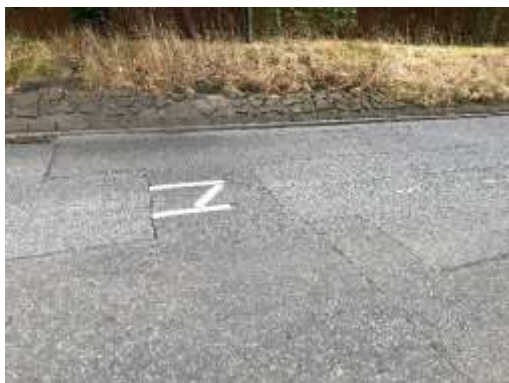
Southbound (Looking East) – chainage 0
