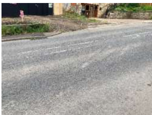
Eastbound (Looking NWW) – chainage 0
