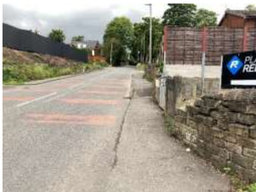
Northbound (Looking North) – chainage 90
