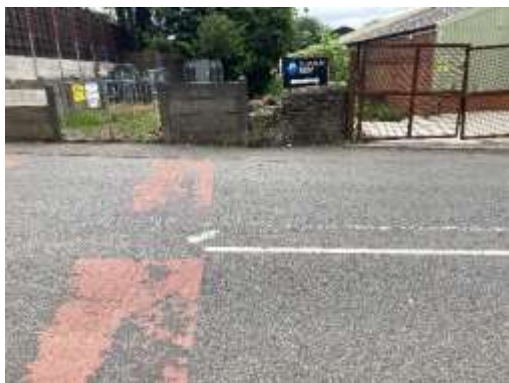
Southbound (Looking East) – chainage 90
