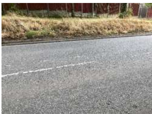
Southbound (Looking East) – chainage 20
