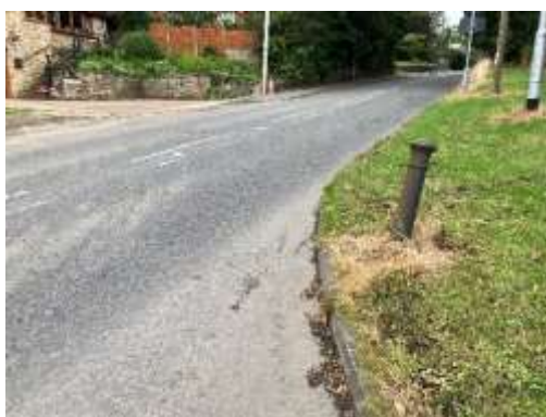
Eastbound (Looking NW) – chainage 0
