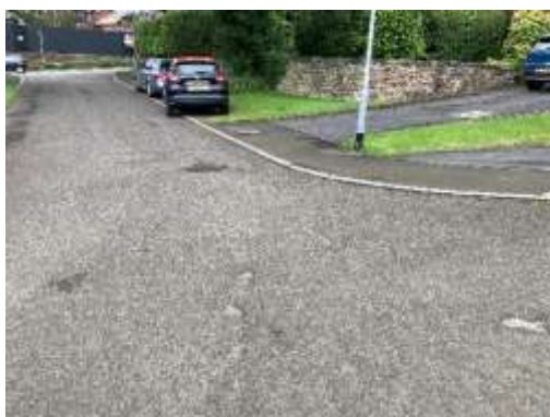
Eastbound (Looking NW) – chainage 40
