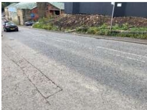
Eastbound (Looking SW) – chainage 0
