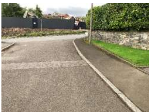
Eastbound (Looking West) – chainage 25
