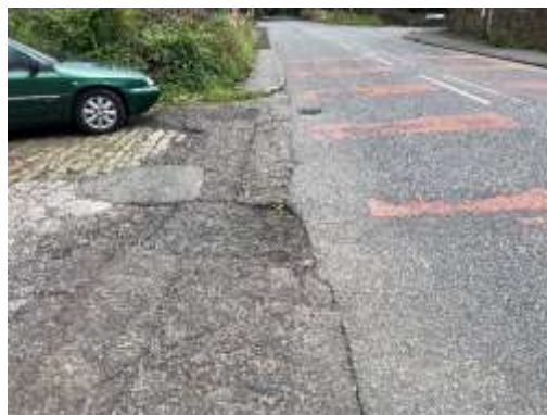
Southbound (Looking North) – chainage 85
