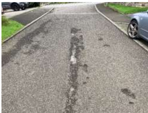
Eastbound (Looking West) – chainage 30
