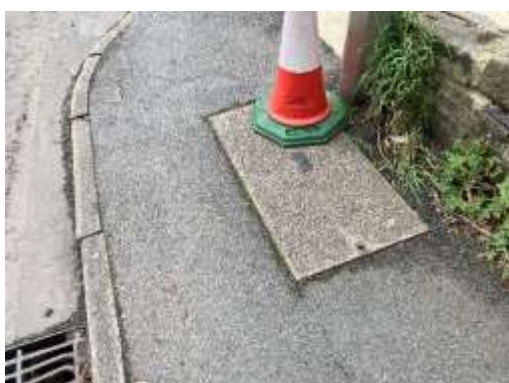
Southbound (Looking Down) – chainage 25
