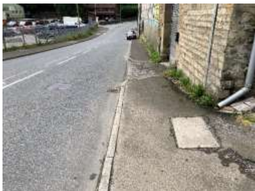
Southbound (Looking South) – chainage 85
