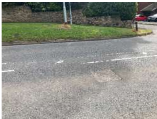
Southbound (Looking East)– chainage 30
