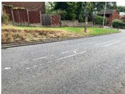
Southbound (Looking SE) – chainage 20
