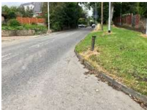
Eastbound (Looking NW) – chainage 3
