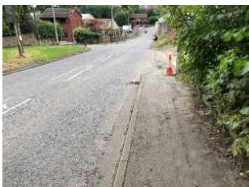
Southbound (Looking South) – chainage 20
