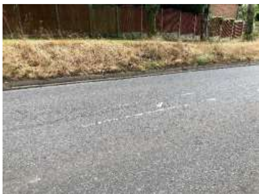
Southbound (Looking East) – chainage 10
