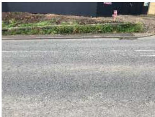
Eastbound (Looking West) – chainage 0
