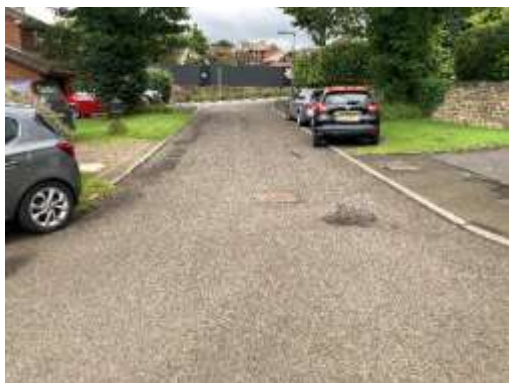
Eastbound (Looking West) – chainage 40
