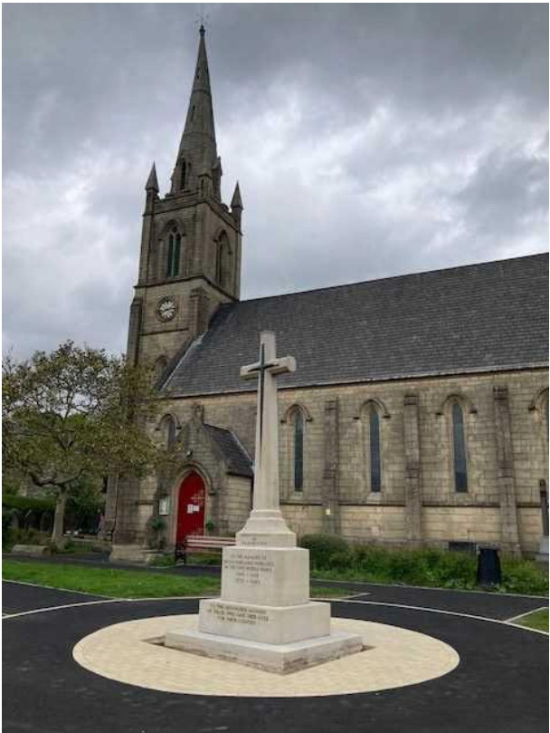
Figure 6 – Church of St Paul, Grade II (background) War Memorial, Grade II (foreground)
