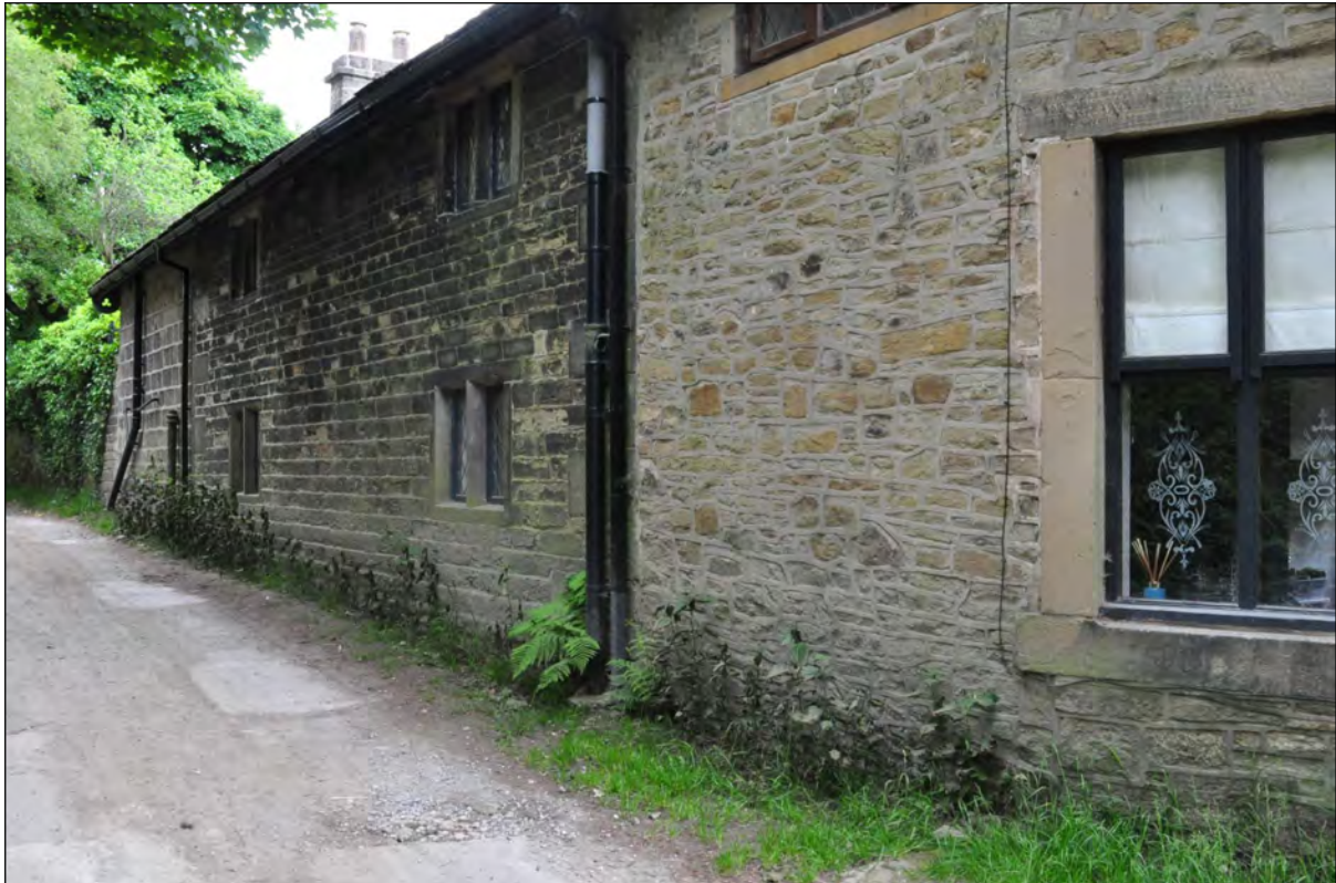
Photo 3: Rear of house, looking east along Moorbottom Road
