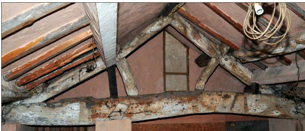
Photo 10: South roof truss in barn. Tie-beam is re-used cruck
