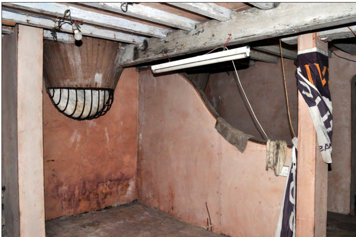
Photo 9: Stable (former shippon) in south end of barn
