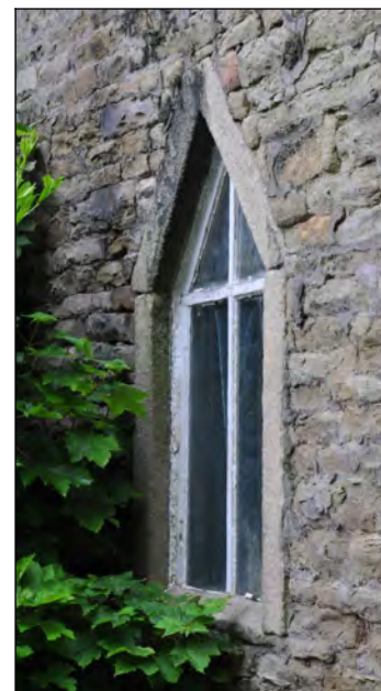
Photo 8: Arched window in south side of barn
