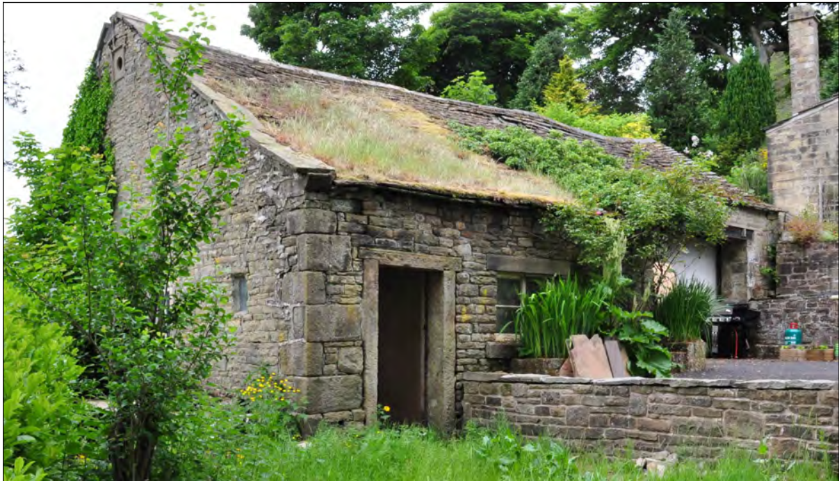
Photo 6: Barn, looking north-west
