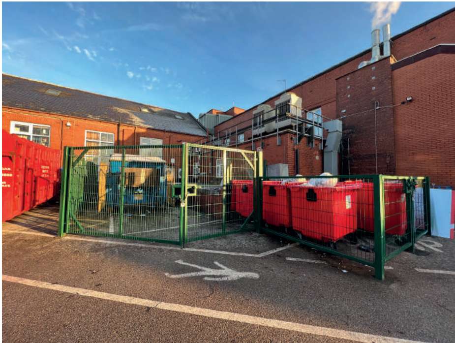
View of the waste storage area from the south
