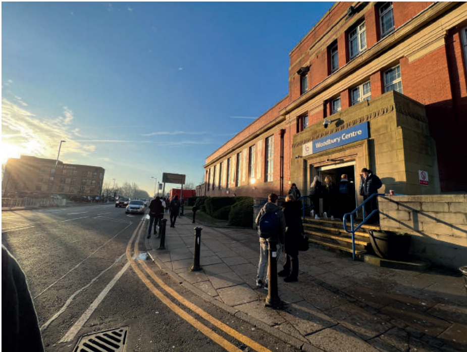
View of the existing main entrance to the Woodbury Centre
