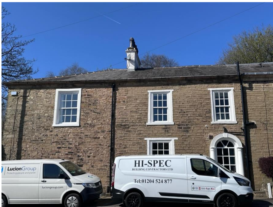
Fig .1, Barwood House
